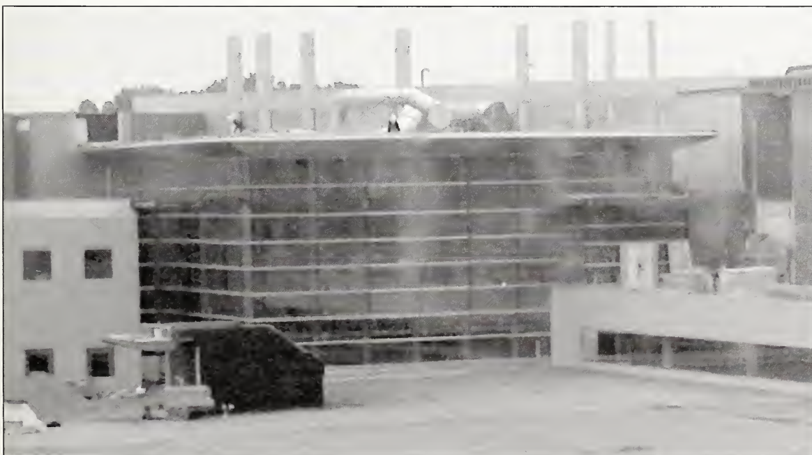
Construction of the AML Cleanroom, late October 2002.
