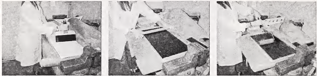
FRP sheet being pressed with trowel
