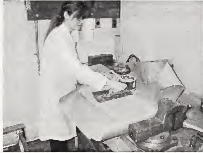
Fig. 5.8 Application of MBrace putty
