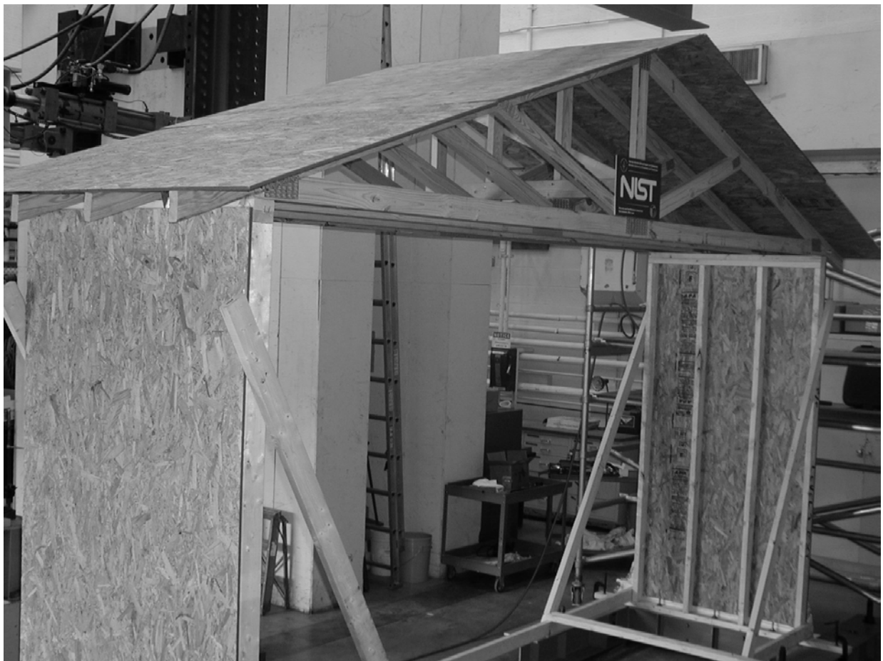
Figure 2.2. Typical test specimen before instrumentation.
