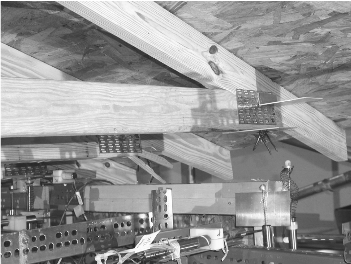
Figure 4.1. Failure of toe-nailed connection with lateral load.
