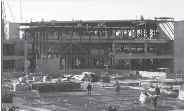
Construction of the AML Cleanroom, late Oct. 2001.
