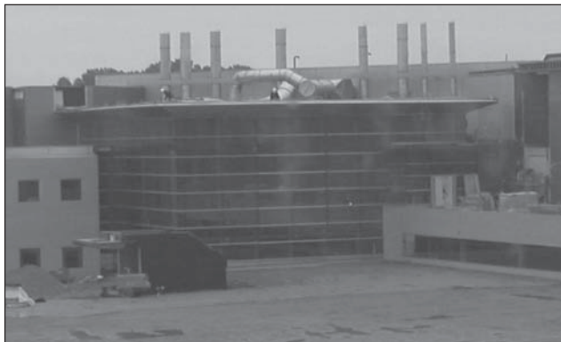
Construction of the AML Cleanroom, late Oct. 2002.
