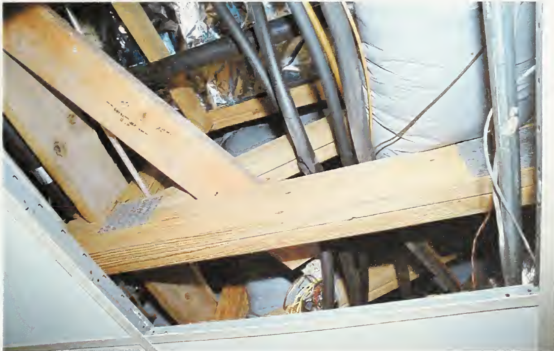
Figure 5. Attic area in a similar restaurant showing the trusses.
