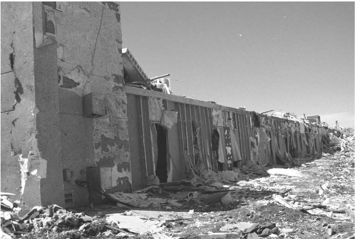
Figure 3-7: Damage to North Side of the Hampton Inn.
