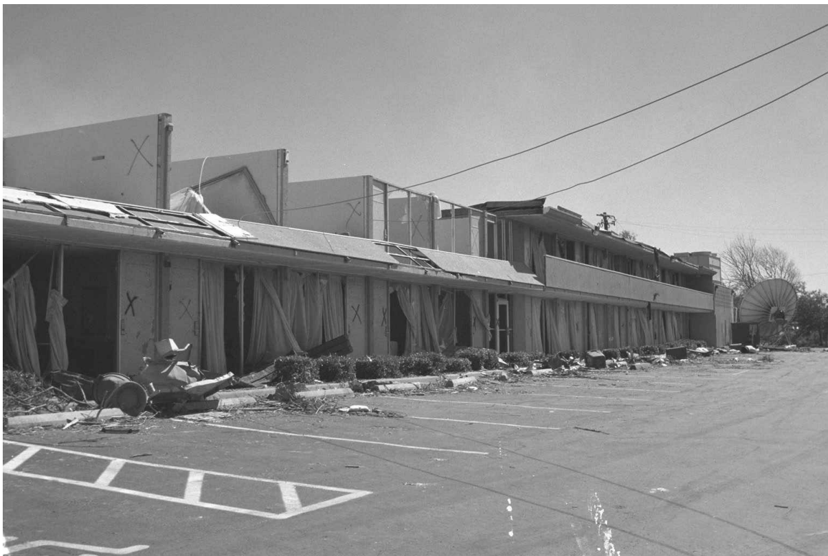
Figure 3-2: Damage to South Side of the Clarion Inn.
