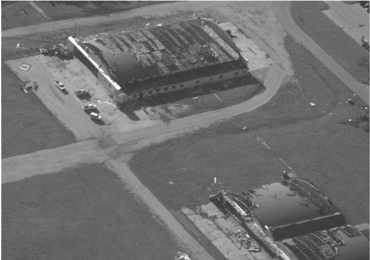
Figure 5-1: Aerial View of Damage to Hangars at Chickasha Airport
