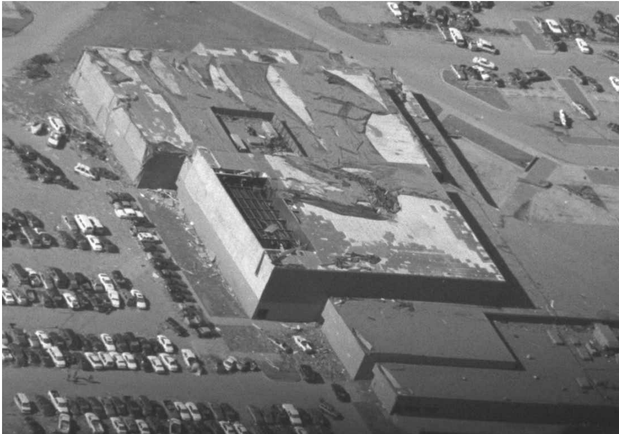
Figure 2-13: Detail of Roof Damage to Westmoore High School.
