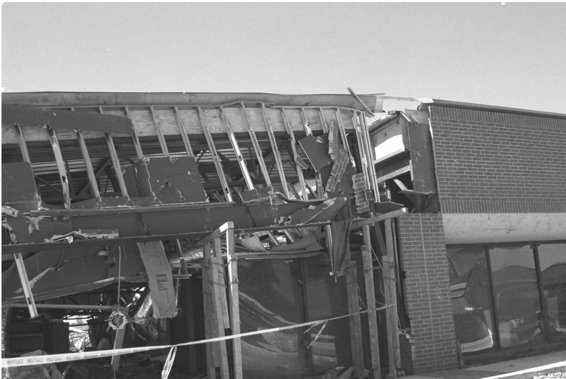
Figure 4-4: North Side of the South Building at Joint between Sections.
