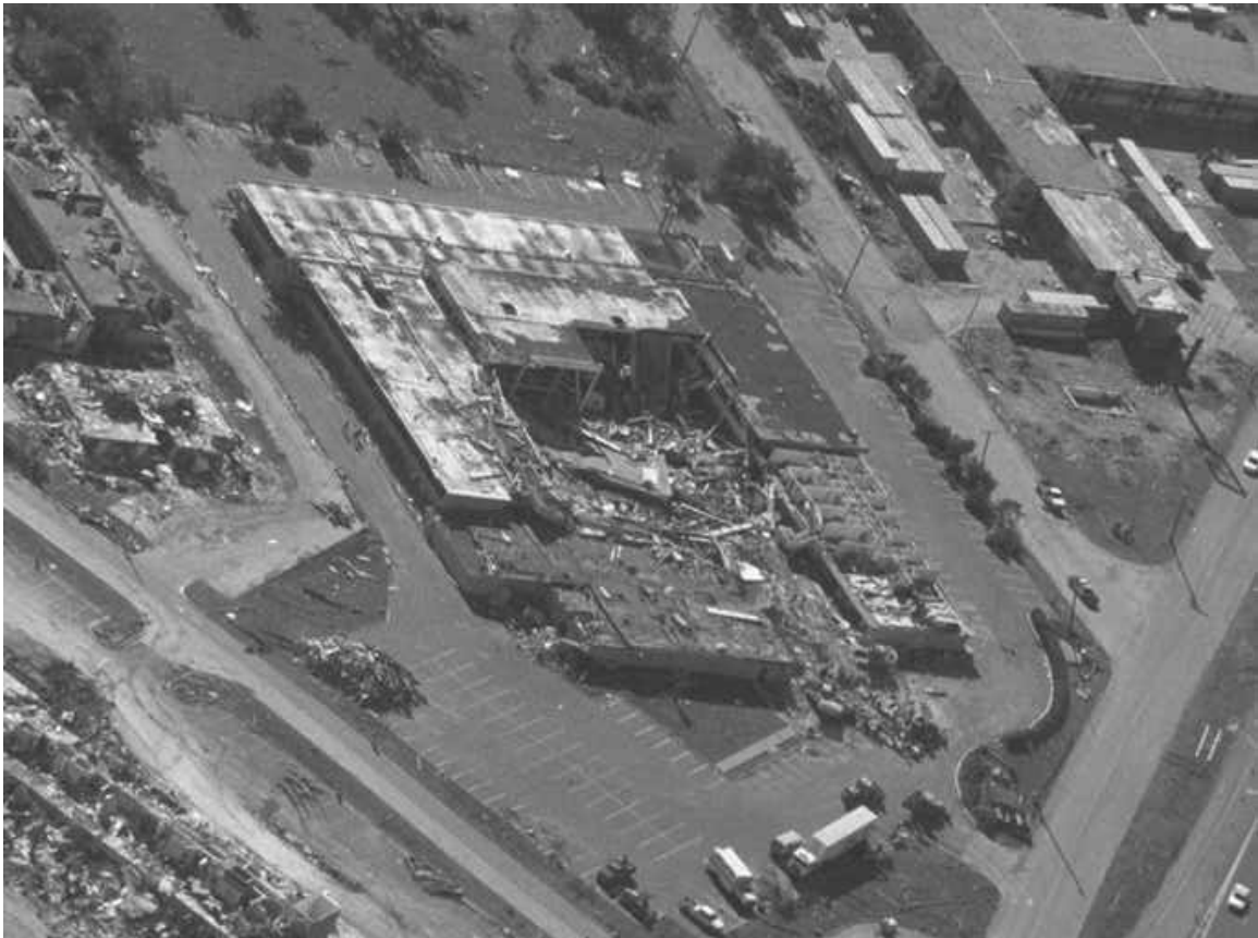
Figure 3-1: Aerial View of Damage to the Clarion Inn.
