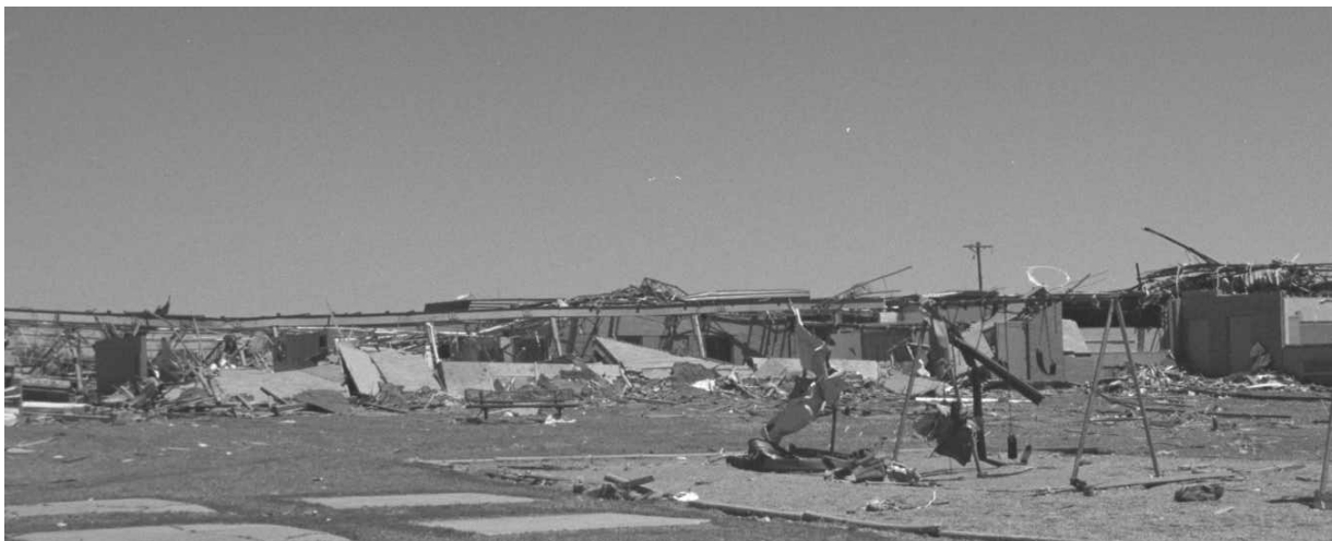
Figure 2-4: South Side of the Center Section of Kelly Elementary School.
