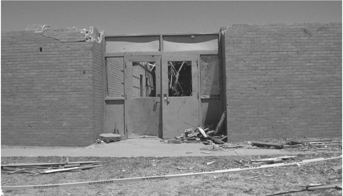
Figure 2-6: South Side of the East Section of Kelly Elementary School.
