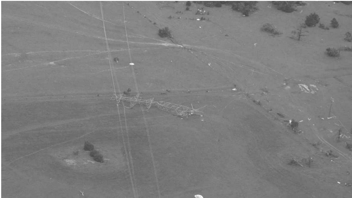
Figure 5-5: Destroyed Transmission Tower near Crescent, Oklahoma.
