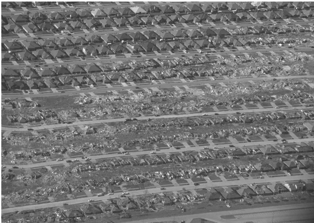
Figure 1-4. Damaged Housing Complex South of Westmoore High School, Oklahoma City.
