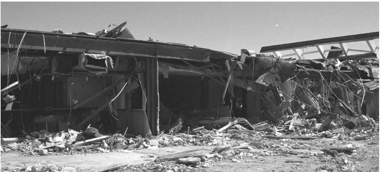
Figure 3-4: Damage to Western Section of the Clarion Inn.
