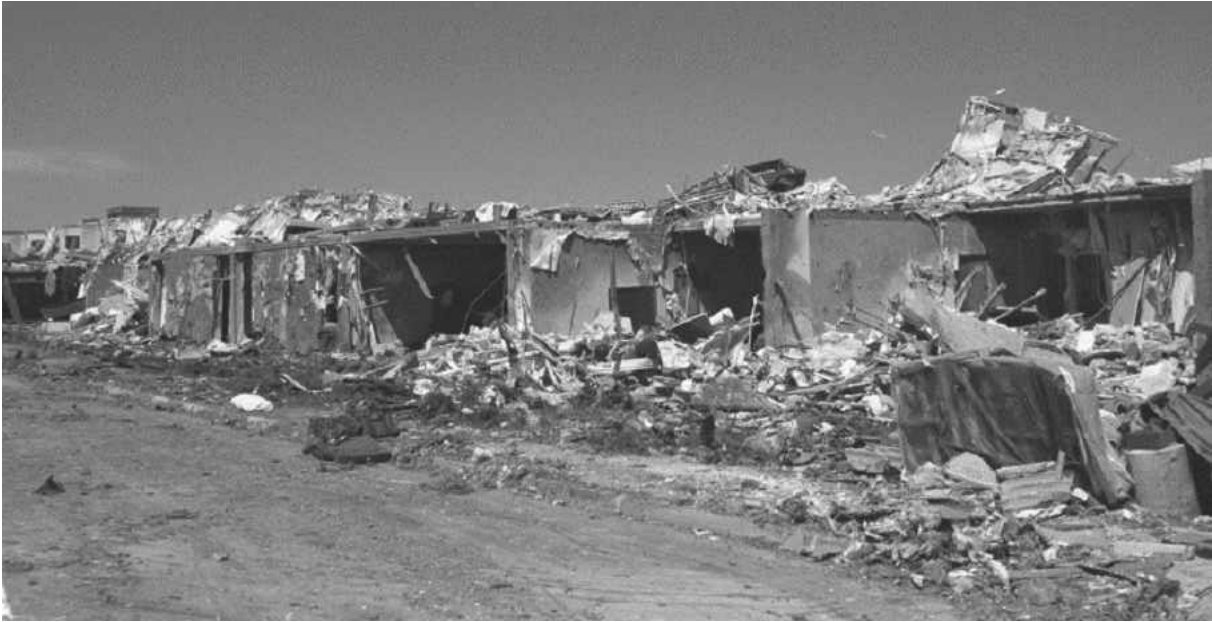
Figure 3-6: Damage to South Side of the Hampton Inn.
