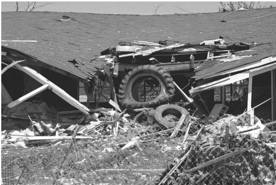
Figure 5-3: Debris Damage to Building Adjacent to Regency Park Baptist Church.
