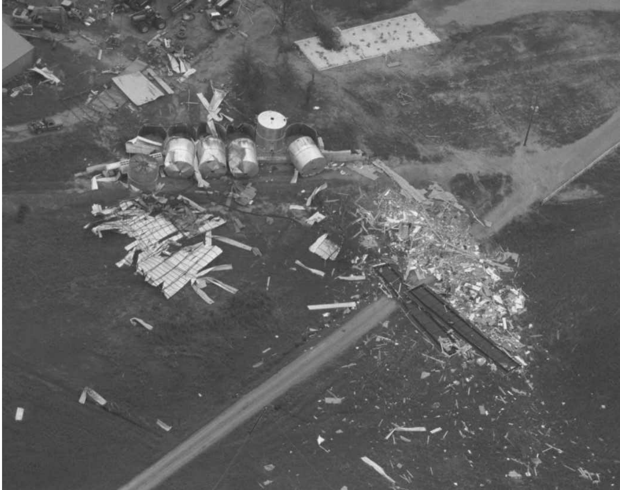
Figure 5-7: Damage to Farm buildings and Silos near Crescent, Oklahoma.
