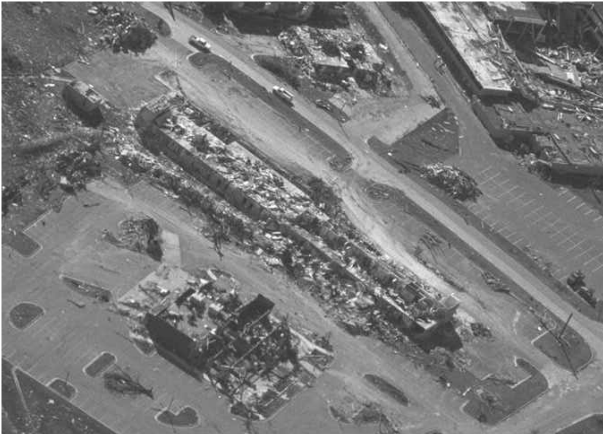
Figure 3-5: Aerial View of Damage to the Hampton Inn (long rectangular building).
