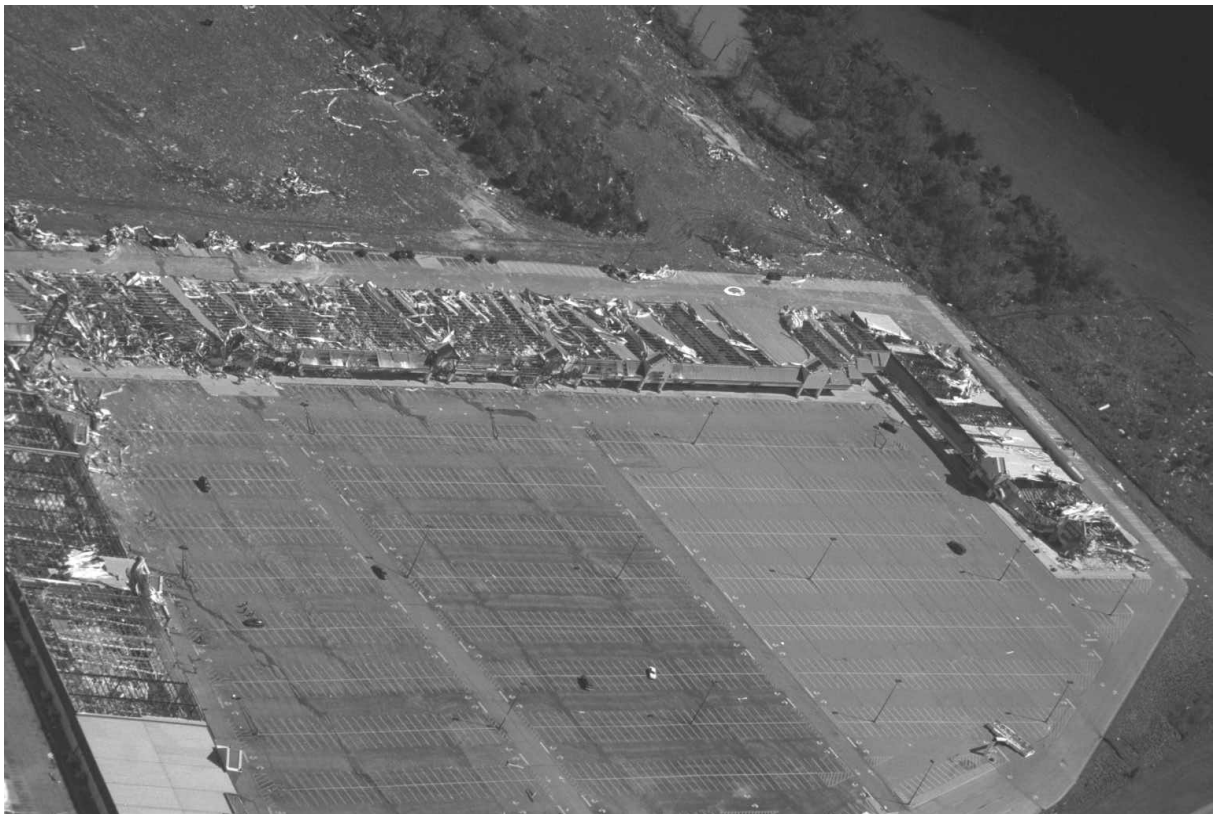
Figure 5-4: Aerial View of Damage to the Tanger Outlet Center Mall.
