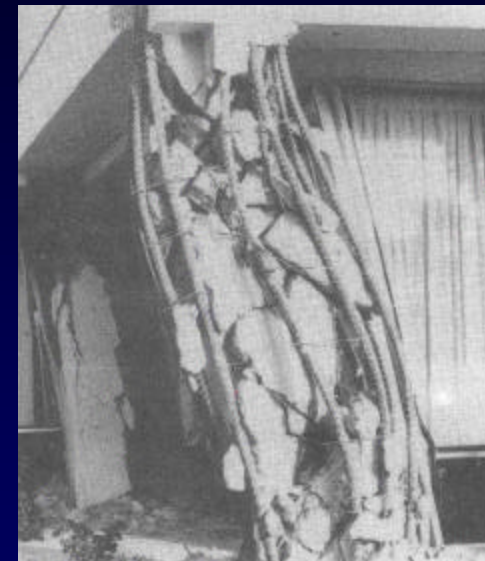
Column Failure
