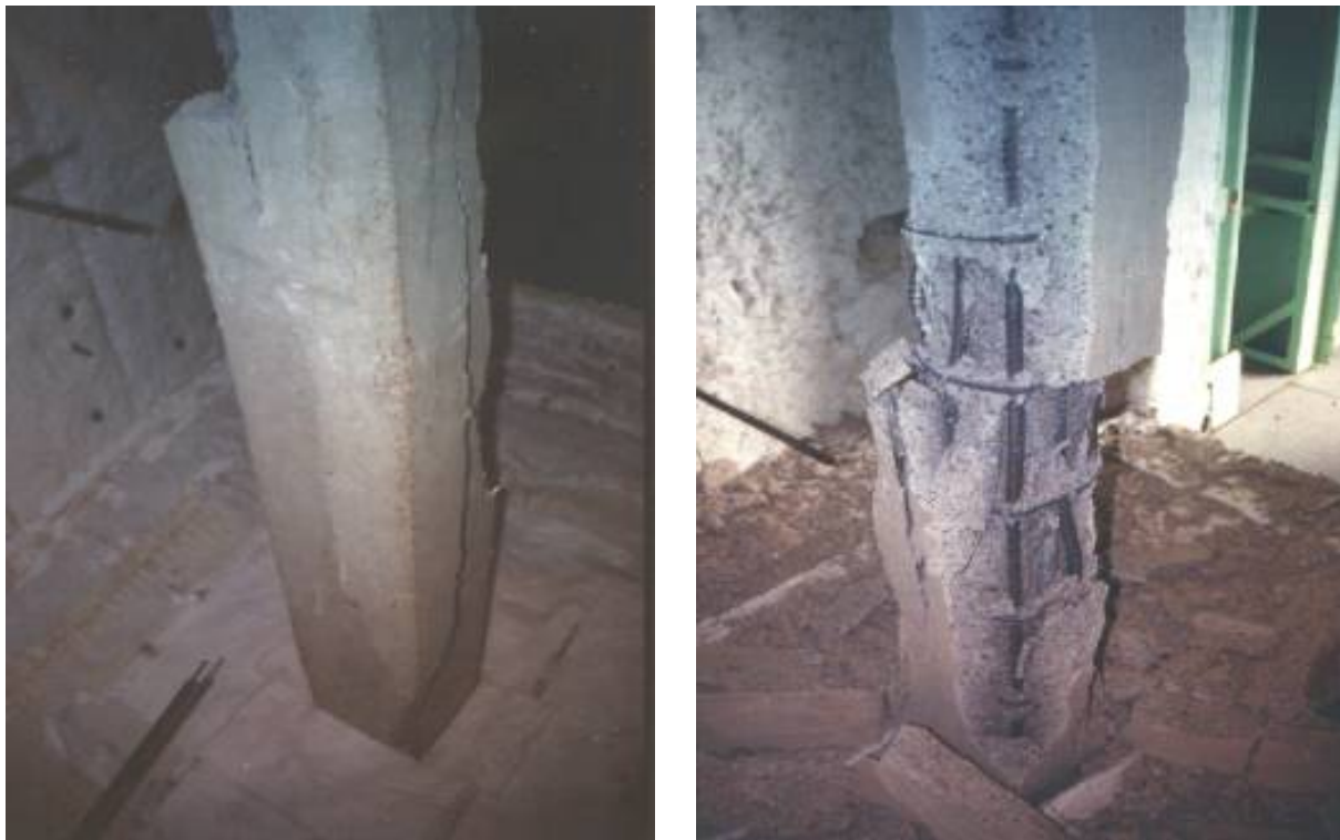
Figure 5. Comparison between normal strength concrete (left) and high strength concrete (right) after ASTM E119 column test.
