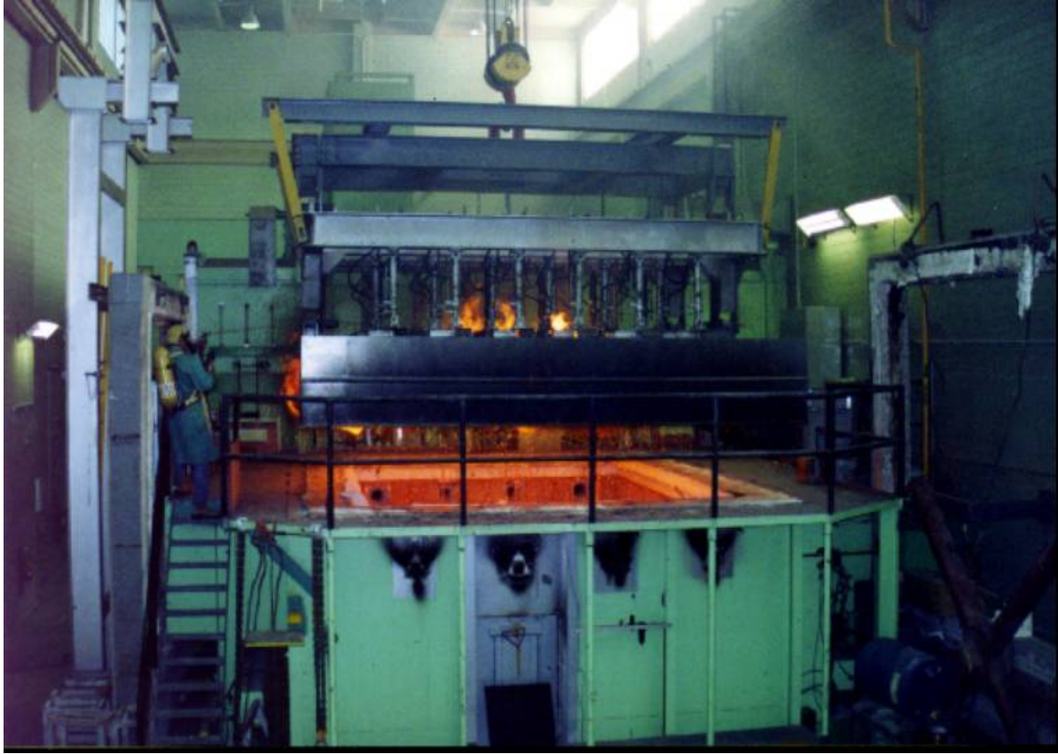
Figure 6. Photograph of modern floor testing furnace (Kodur)
