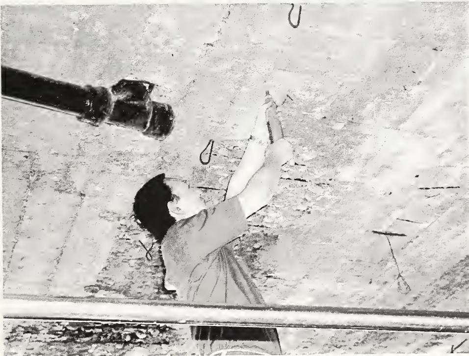
Bottom of Second Floor Slab.
