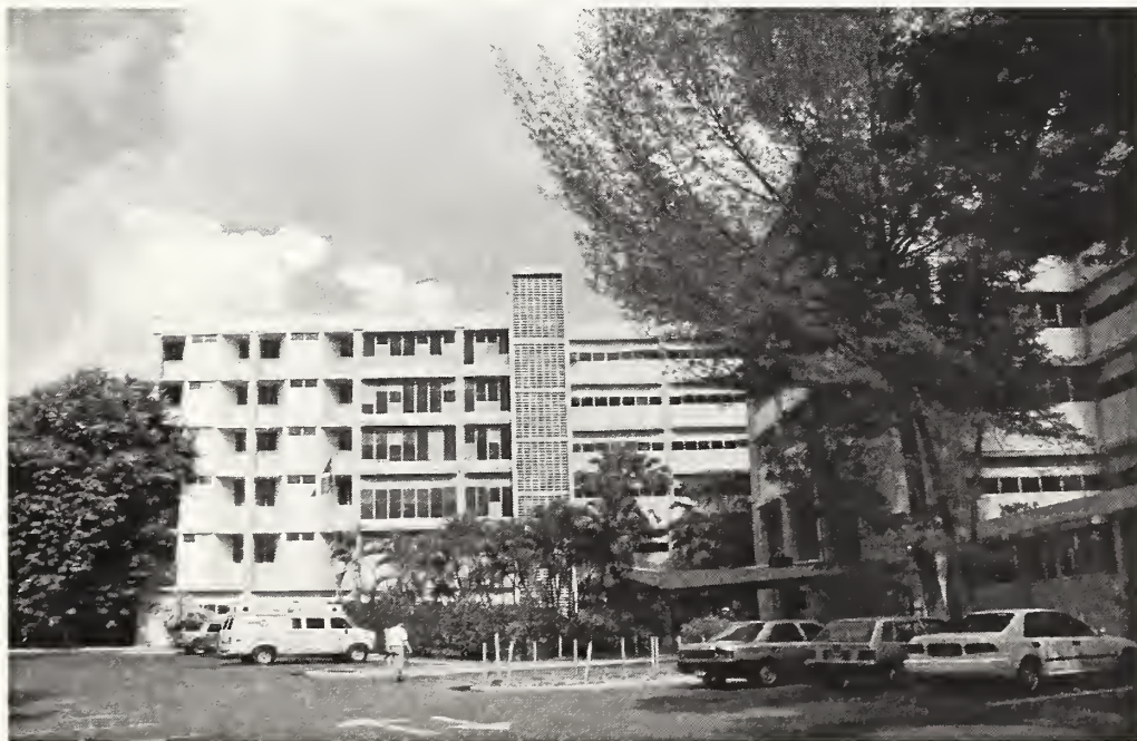
South Wing of Hospital
