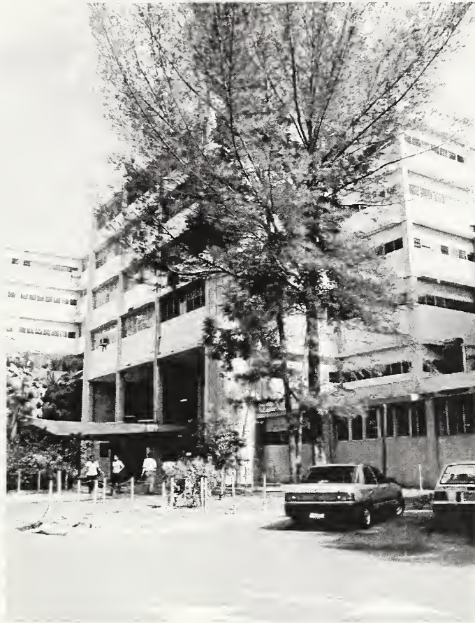
View from the rear of Hospital
