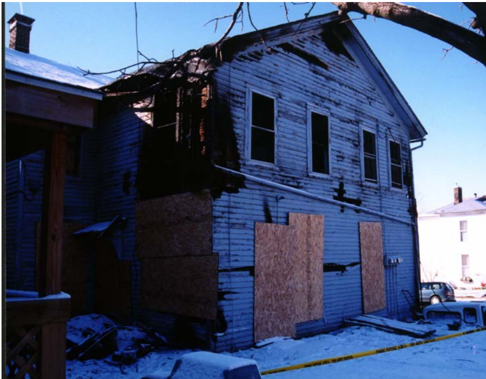
Figure 2. Back of structure.
