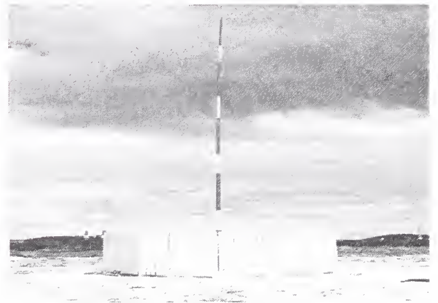
Figure 8. New whip antenna at WWVH on Kauai. Conventional antennas are seen in the background. The fencing is a safety measure, preventing personnel access to the high voltages on the antenna system.
