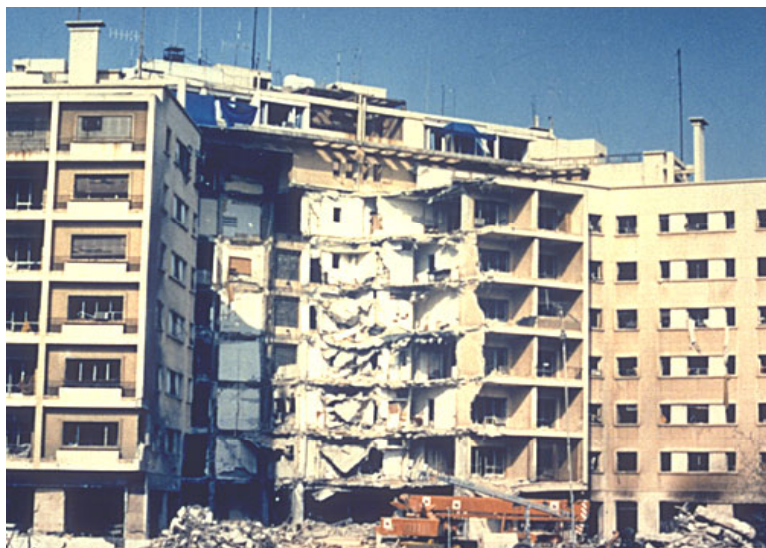
Fig. 1— Example of progressive collapse initiated by ground level blast loading.
