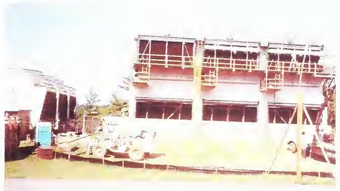
Fig. 2. The new plume-abated cooling tower (right) nears completion. It will replace the lower capacity and less efficient system that had no abatement ability (left).
