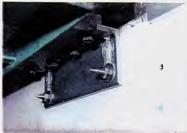
LT: Lift table attachment at thermal column
