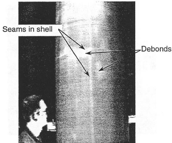
*Figure 3. Debonds in a prefabricated shell.*
