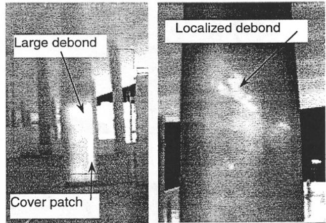
*Figure 4. Large debond in a pre-fabricated shell*
