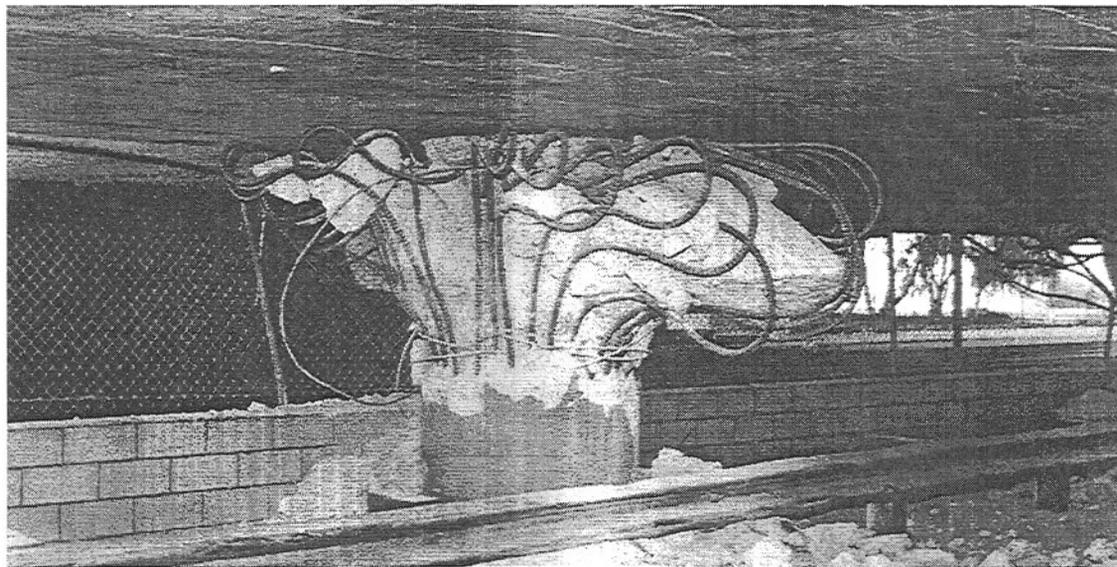
**FIG. 1. Progressive Shear Failure, I-10 Santa Monica Freeway,
