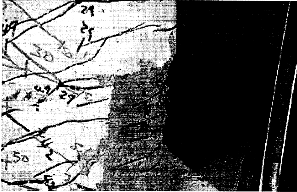
FIGURE 5-13 Final Damaged State of Specimen A9
