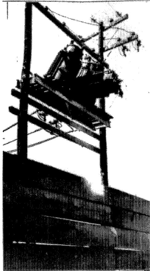
Figure 15. Fallen platform-mounted distribution transformer in the 1952 Kern County, California, earthquake.
