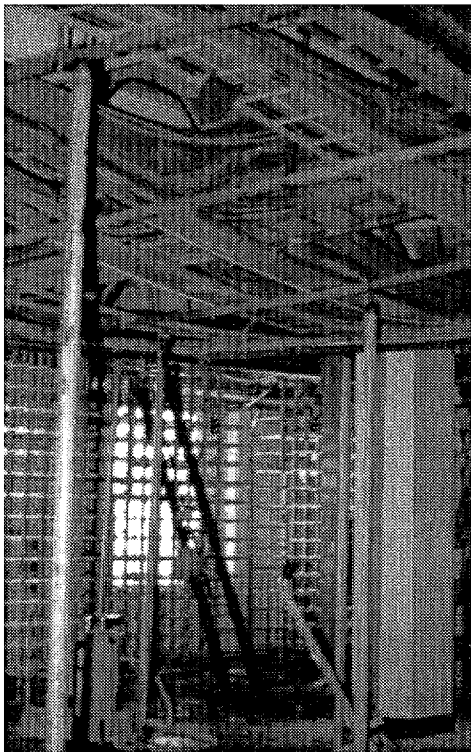
Photo 6. Ironwork failure during Whittier Narrows earthquake in 1987. Note the friction clips used.
