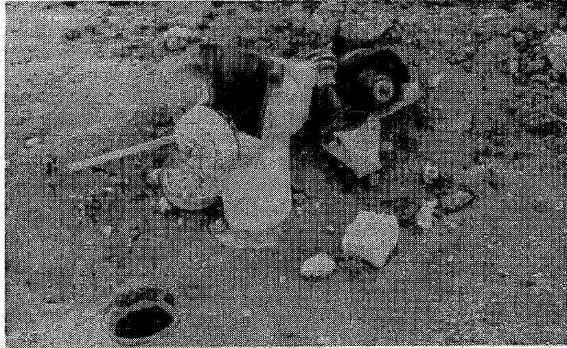
Figure 13. This water hydrant was shattered by the high water pressures generated during the 1971 San Fernando, California, earthquake. The pressures were presumably the result of underground deformations of pipes caused by soil strains. Such damage to the water supply system makes a community vulnerable to uncontrolled fires.
