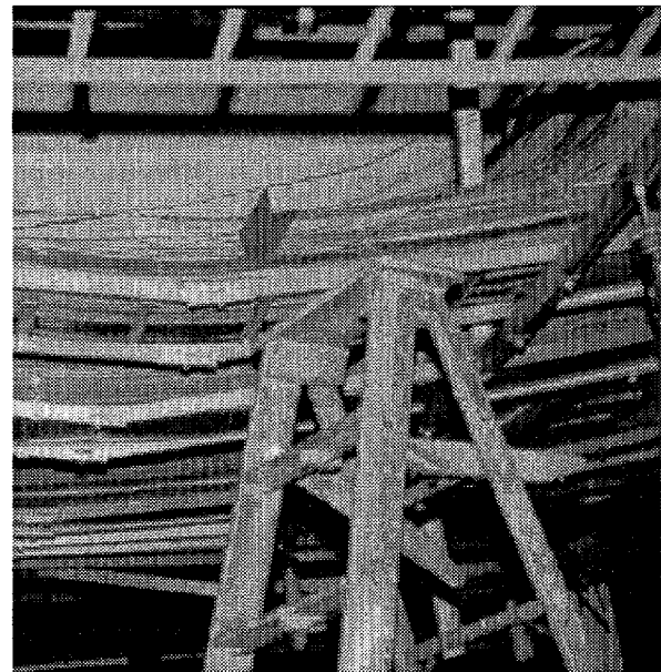
Photo 6. Ironwork failure during Whittier Narrows earthquake in 1987. Note the friction clips used.
