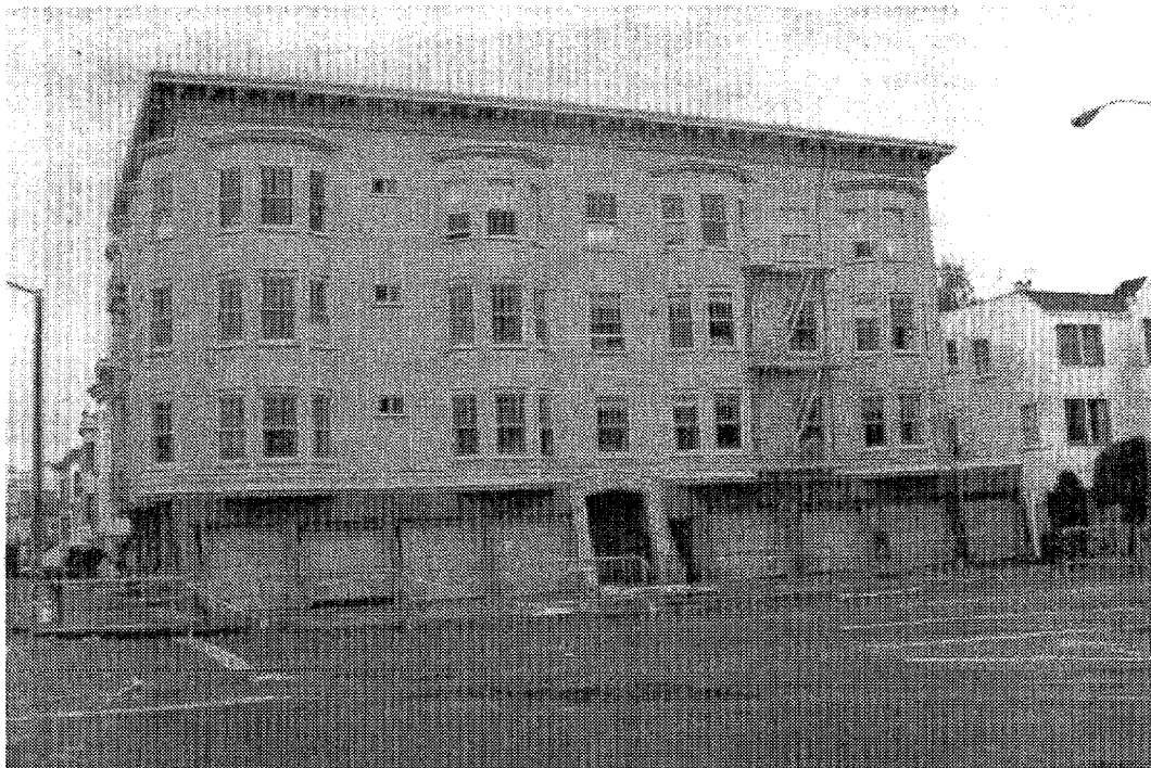
Figure 2b. Example of four-story building with multiple garages in the first story (location #1).
