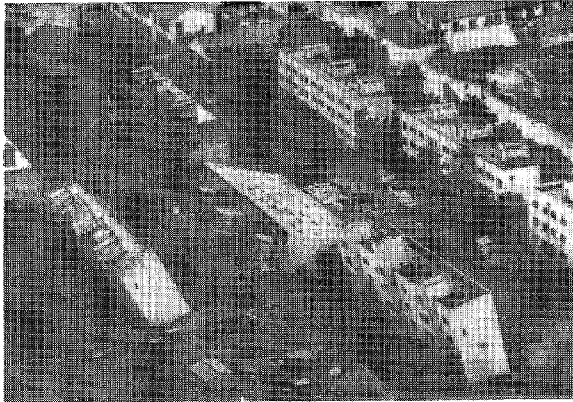
Figure 3a. Tilting and settlement of apartment buildings in Niigata, Japan, because of liquefaction of the underlying soil during the 1964 Niigata earthquake. Photograph: Courtesy of G. W. Housner.
