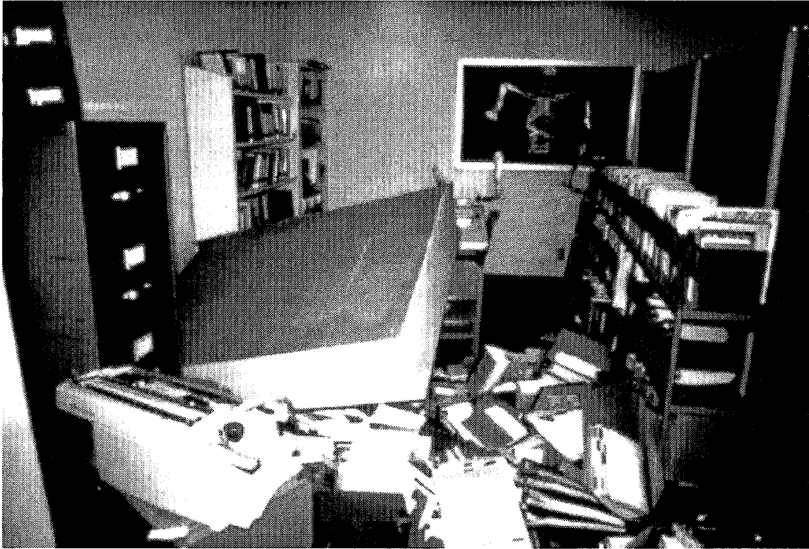
Figure 9. Example of earthquake non-structural damage.
