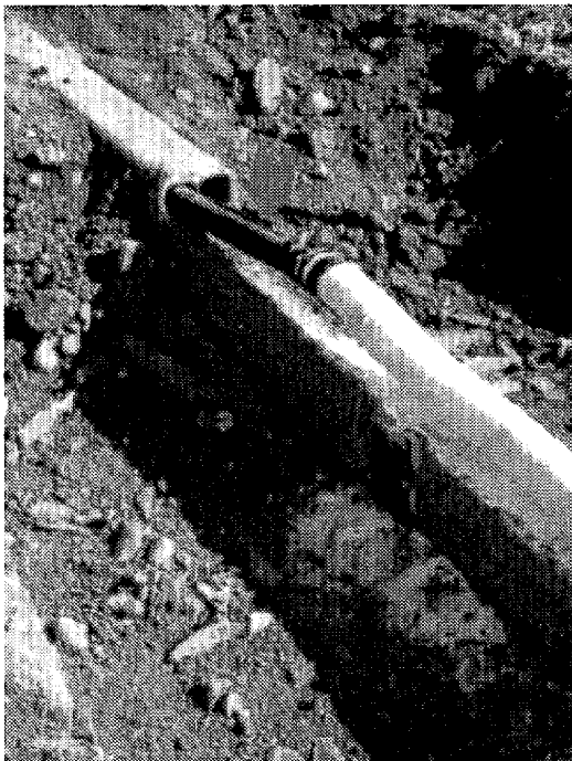
Photo 10. Burying fibre optic cable in process.
