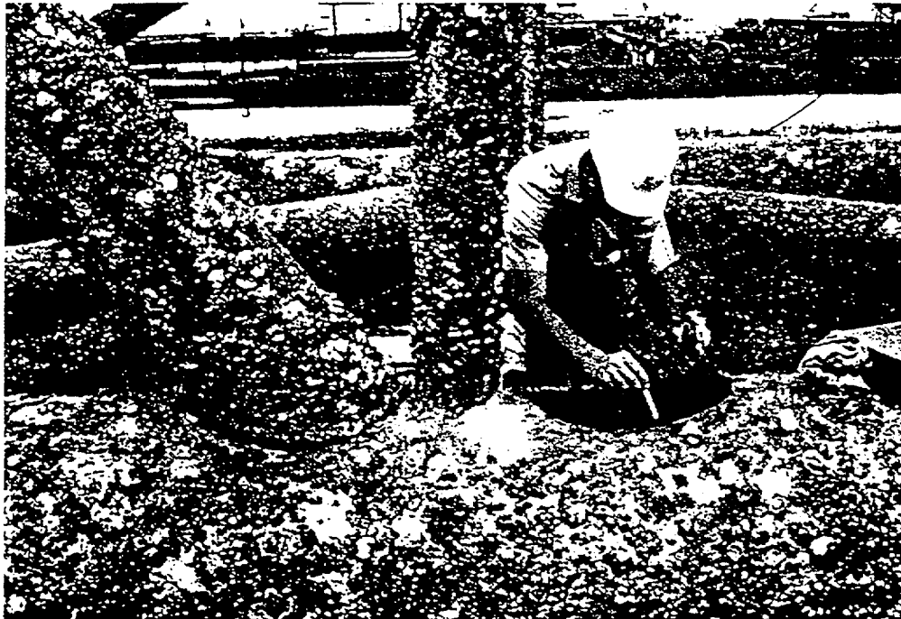
Figure 15: Example of local failure in service
