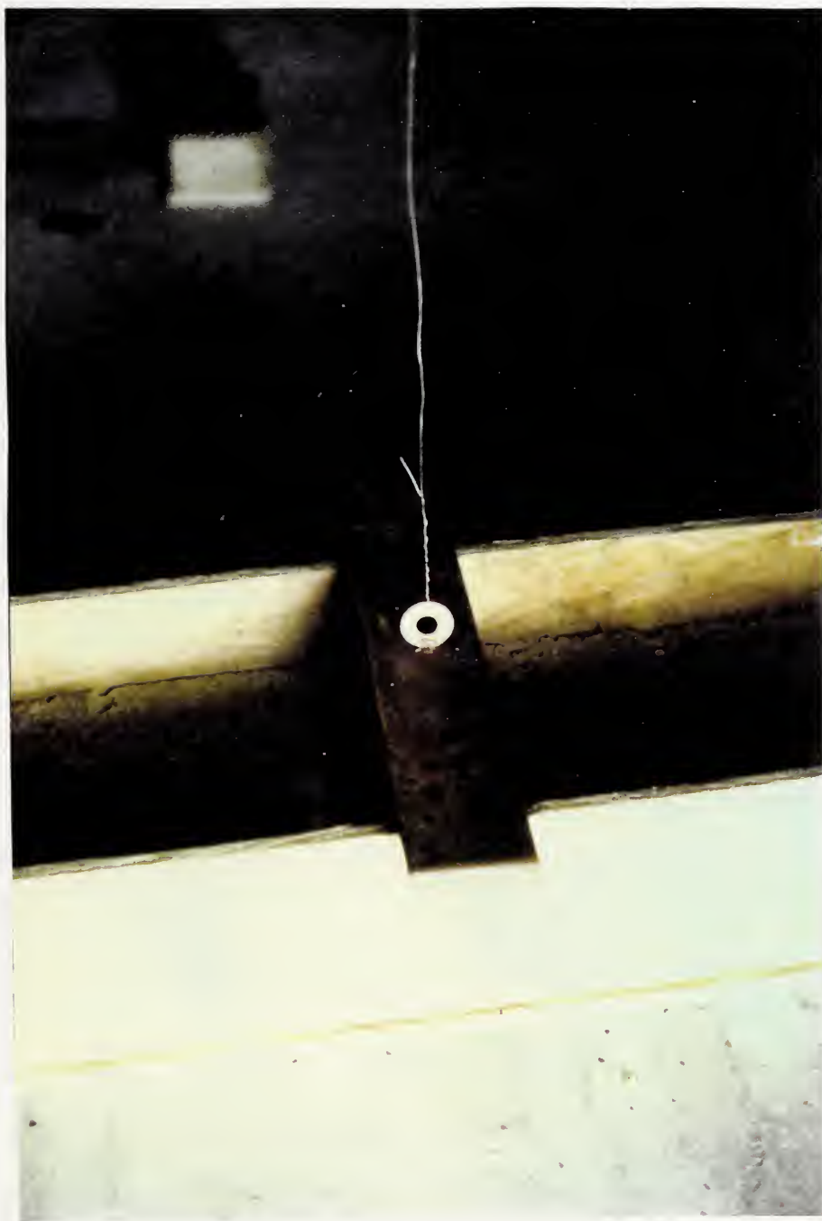
Figure B2. Photograph showing load bearing boxes and deflection gauge weight on purlin
