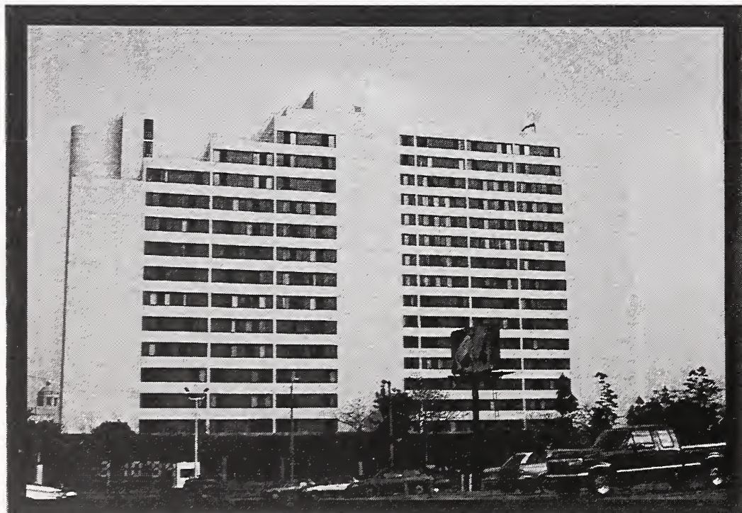
Figure 10 Cathay Manor, a 16-story building about 33 km from the epicenter, was determined to be a concrete shear wall building.
