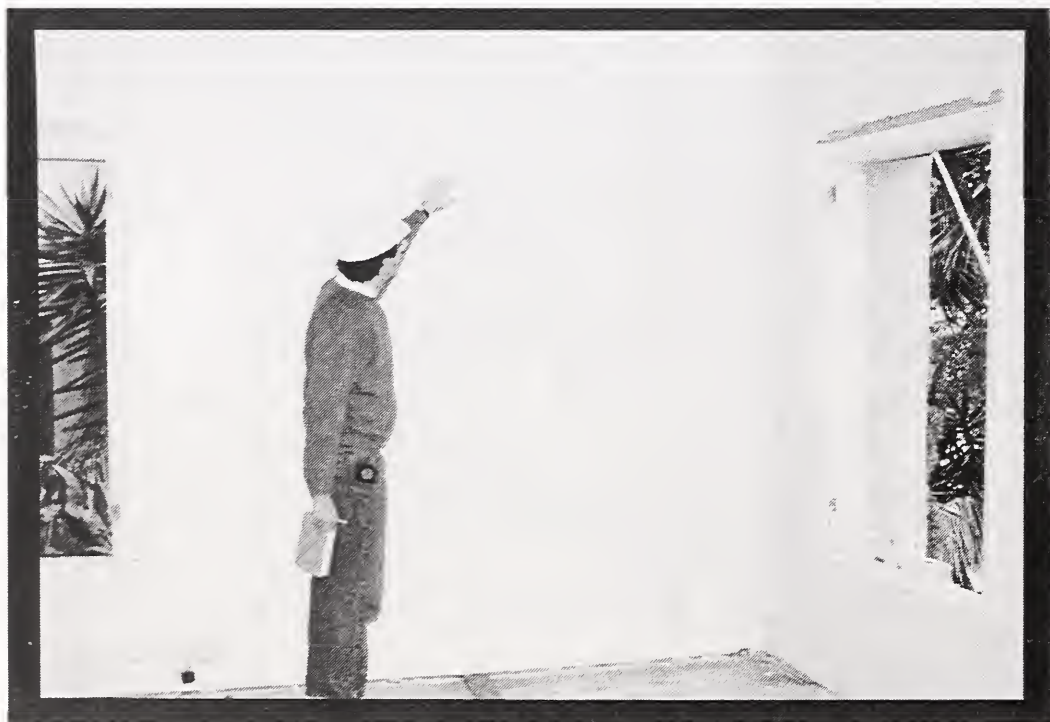
Figure 24 Damage observed in unreinforced masonry buildings included cracks in the interior plaster.
