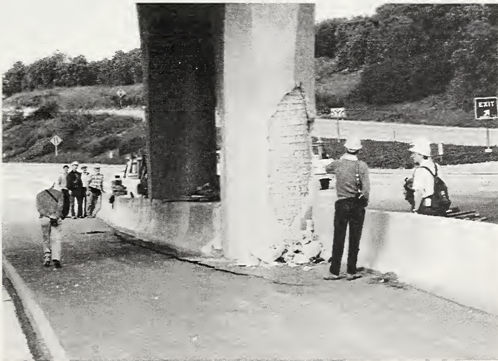
Figure 4.31 SR118 Ruffner Ave. Overcrossing, easternmost central pier, looking to the west
