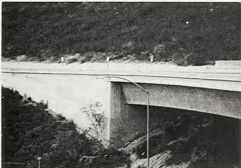
Figure 4.56 Overview of abutment at the east end of the ramp connecting eastbound SR118 with northbound I210
