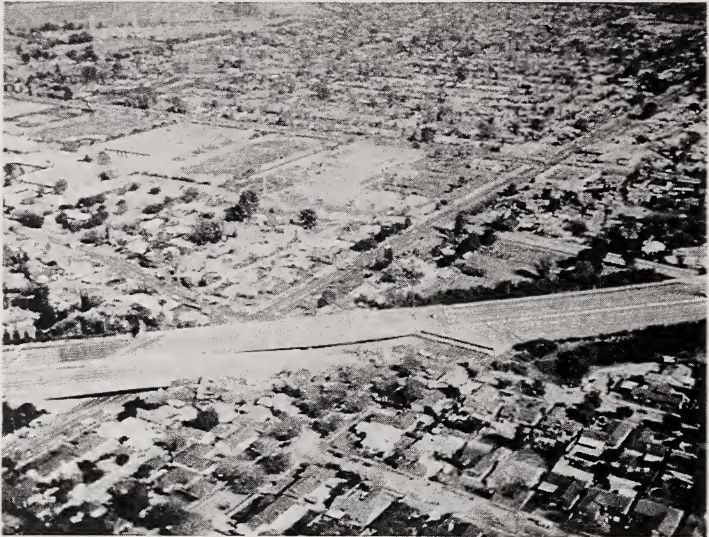
Figure 4.19 Aerial view of the SR118 Mission-Gothic Undercrossing, looking to the north showing collapsed eastbound bridge (Courtesy of FHWA)
