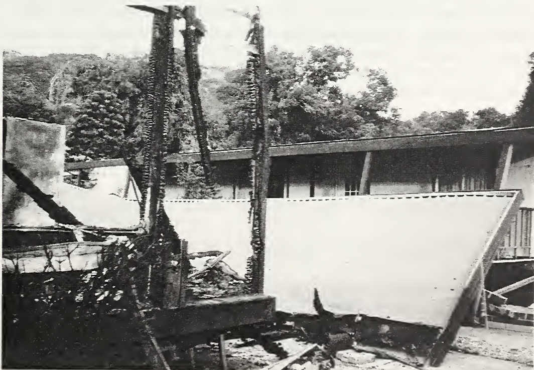
Figure 6.10 Collapsed roof which acted as a fire break in a manufactured housing development.
