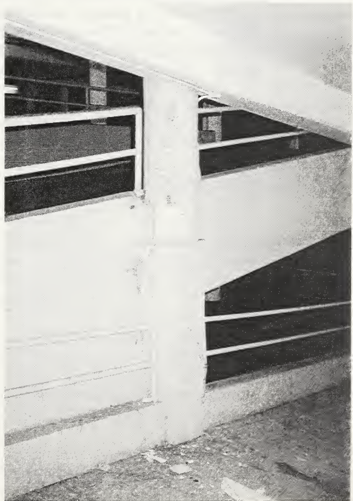
Figure 3.66 At the Northridge Fashion Center, major portions of the three-level south parking garage collapsed. The garage was precast concrete with intermittent shear walls. Most of the shear walls remained standing, largely undamaged, indicating that the lateral load was not adequately transmitted to these walls.
