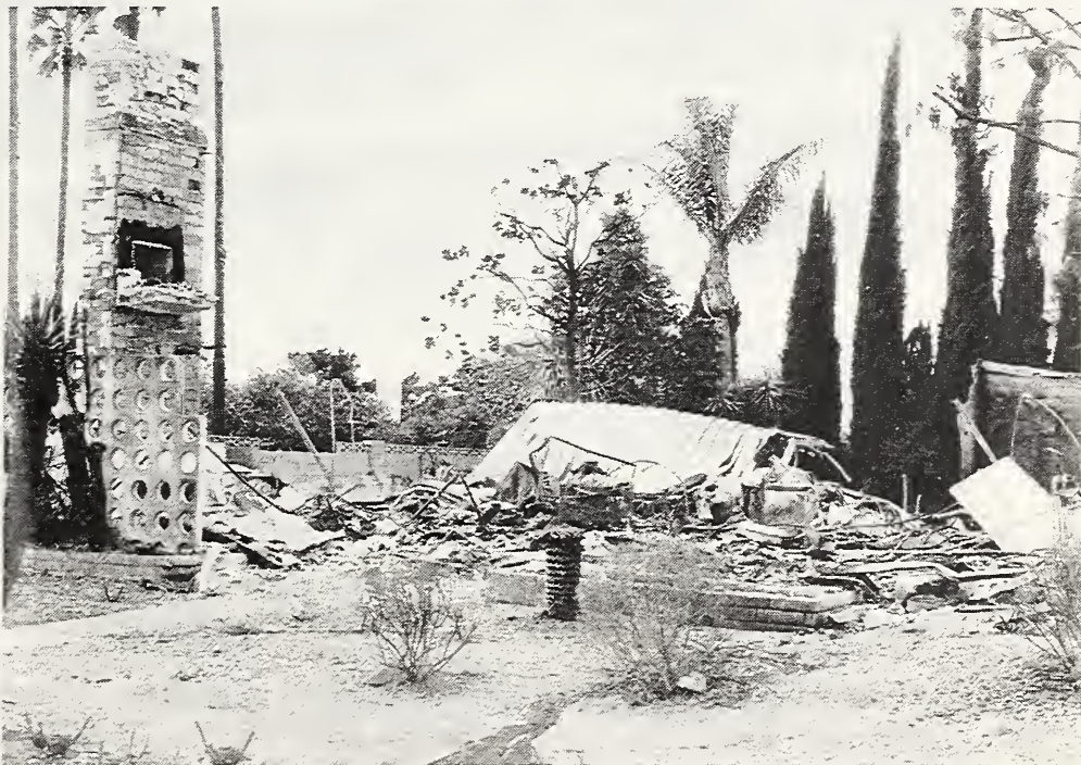
Figure 5.12 Houses destroyed by a fire resulting from the rupture of the 0.6-m gas main along Balboa Boulevard.
