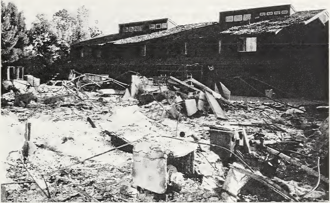
Figure 6.6 Multi-family residential building destroyed by fire.
