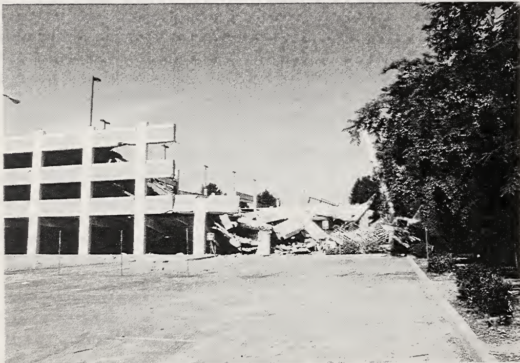
Figure 3.61 Some interior columns of the Northridge campus parking garage remained standing.
