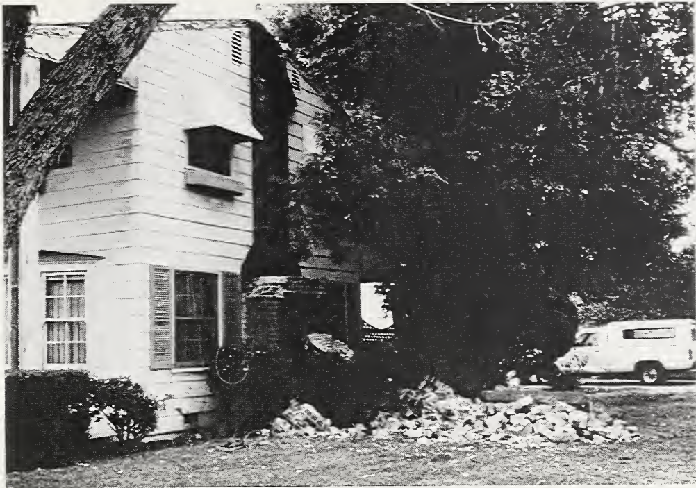
Figure 3.17 Failure of masonry chimneys was common.
