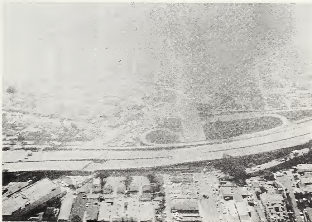
Figure 4.35 Aerial view (looking south) of I10 Separation at La Cienega Blvd. and Venice Blvd., (Courtesy of FHWA)
