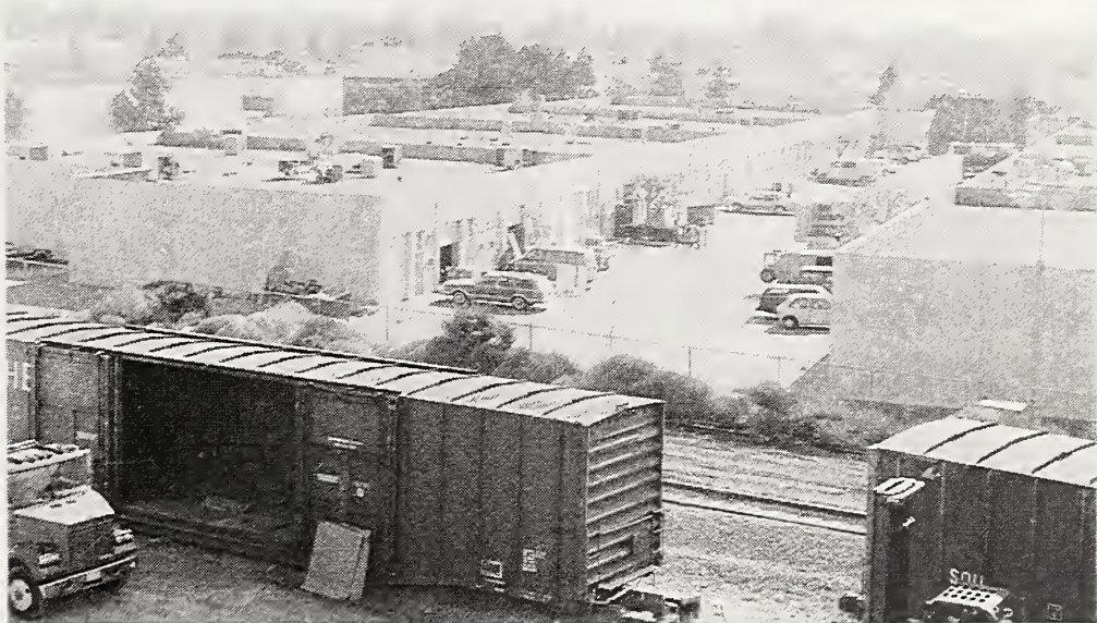
Figure 3.34 The single-story modern masonry commercial buildings directly south of the damaged Levitz furniture store and train derailment were apparently undamaged. All parapets and piers between garage openings appeared intact.
