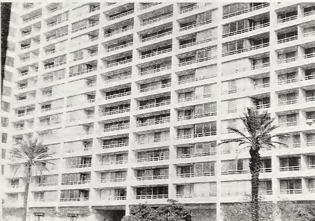
Figure 3.13 The front of the 16-story Champagne Towers building had no apparent damage. Note the steel pipe railings at the balconies.
