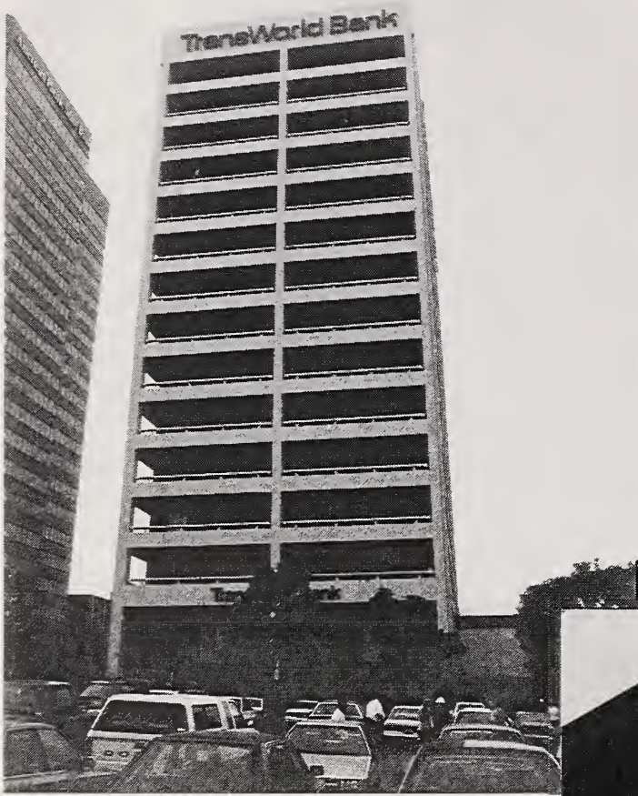
Figure 3.53 The Trans World Bank building, in Sherman Oaks, was damaged in both the 1971 San Fernando and 1994 Northridge earthquakes.
