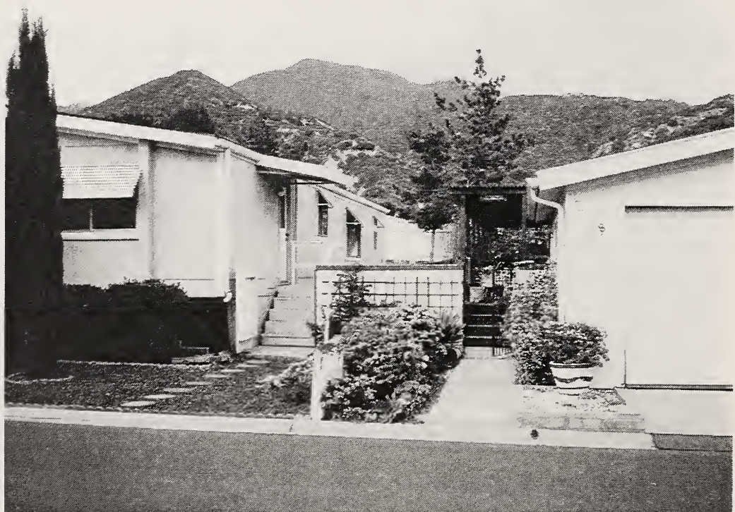
Figure 6.8 Typical unit spacing in a manufactured housing development.
