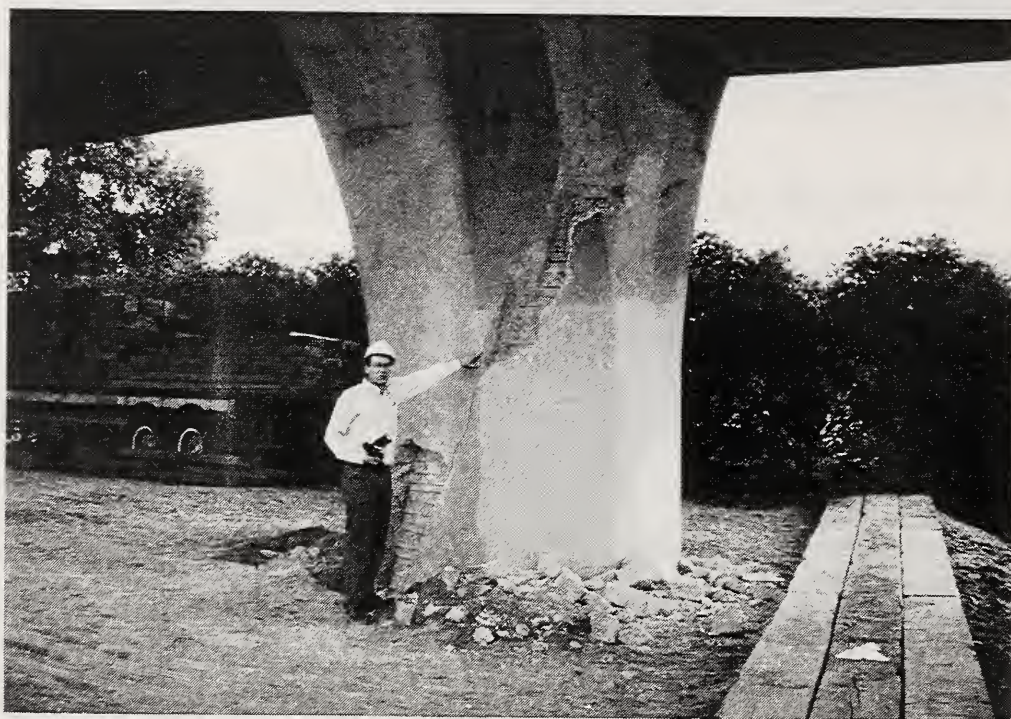
Figure 4.51 View of the westernmost pier at the Interstate 5, State Route 118, Southwest Connector, looking to the southeast. Loose cover concrete has been removed by Caltrans.
