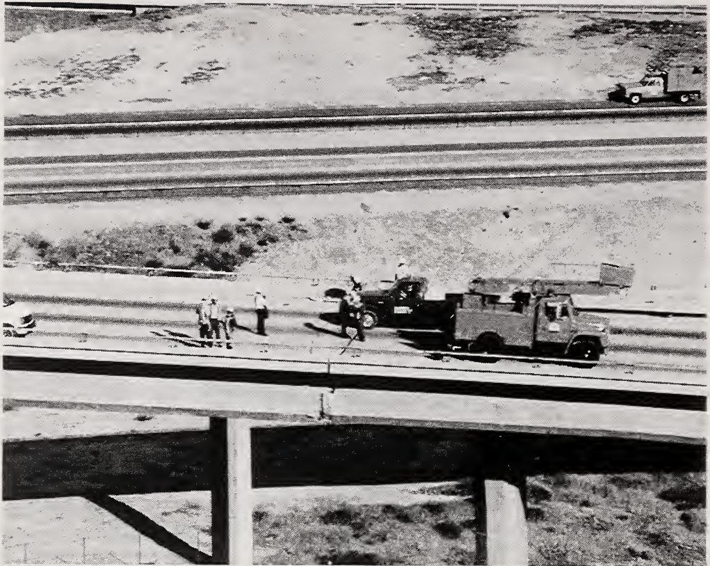
Figure 4.7 Example of pounding and offset at a hinge in the SR14/I5 interchange
