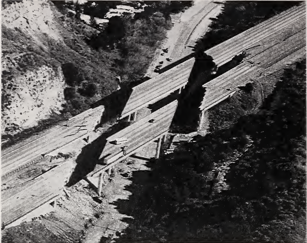
Figure 4.2: Aerial view of the bridge at Gavin Canyon, looking to the east, showing appearance of the four end spans shortly after demolition had begun
