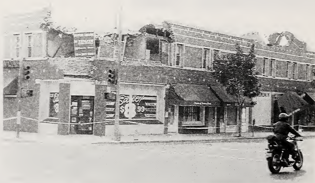
Figure 3.36 Damage to unreinforced masonry buildings, even those that had been rehabilitated, was common. Upper stories and corners were particularly vulnerable to damage. The rows of light-colored diamonds on the face of this building are the end plates of through-bolts used to connect the wall to the floor joists, a typical rehabilitation technique. The remains of parapet braces can be seen on the roof.
