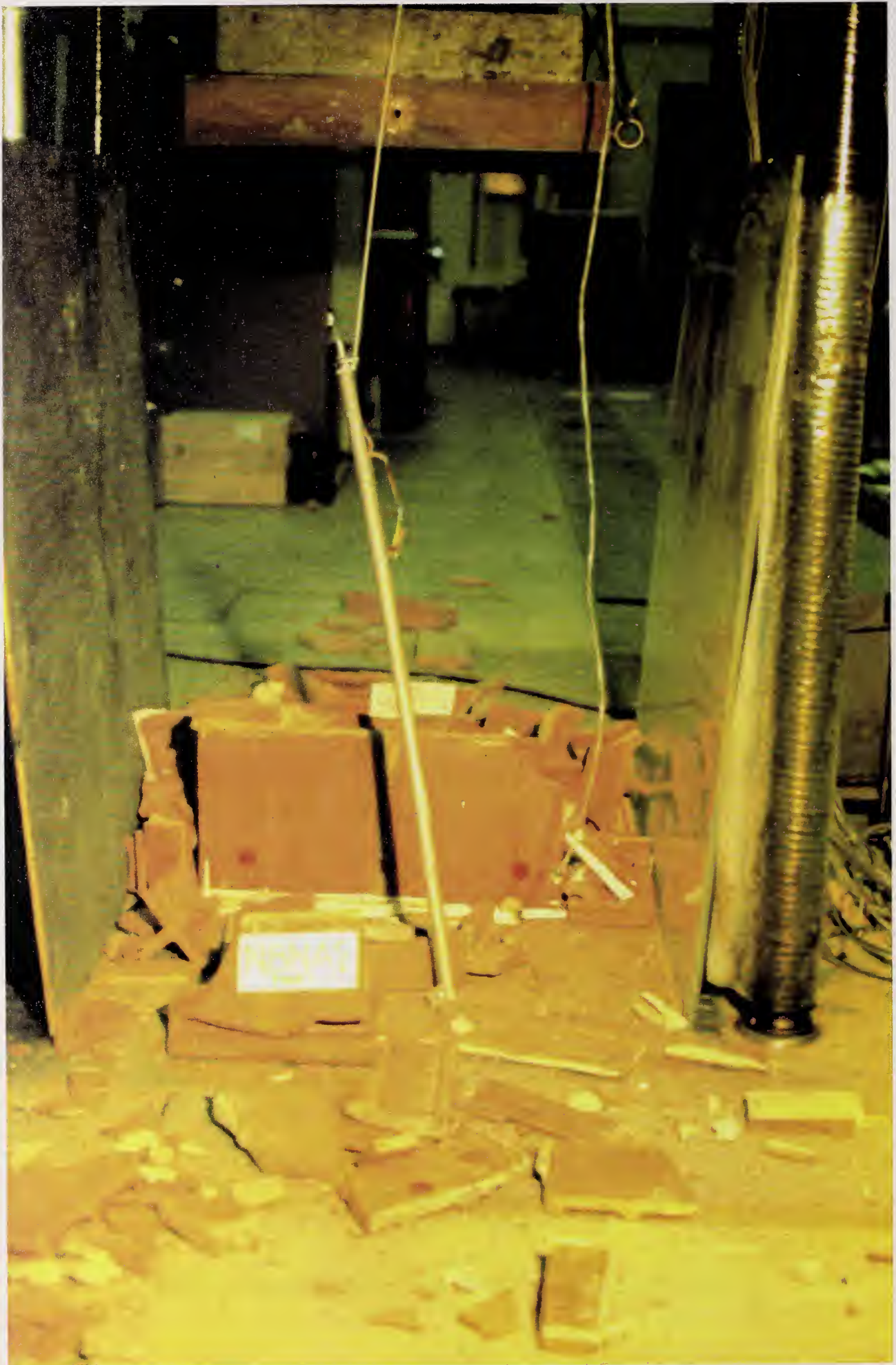
Figure 5.5 - Post Failure View of Typical Normal Prism 44
