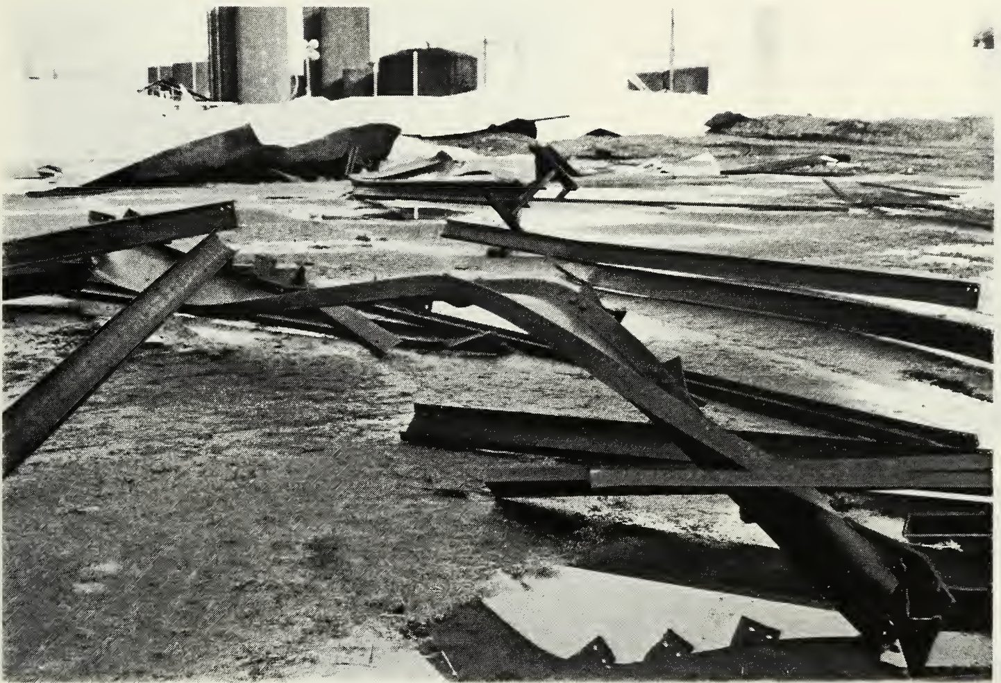
Figure 3.7 - Roof Framing Debris Scattered on Tank Bottom
