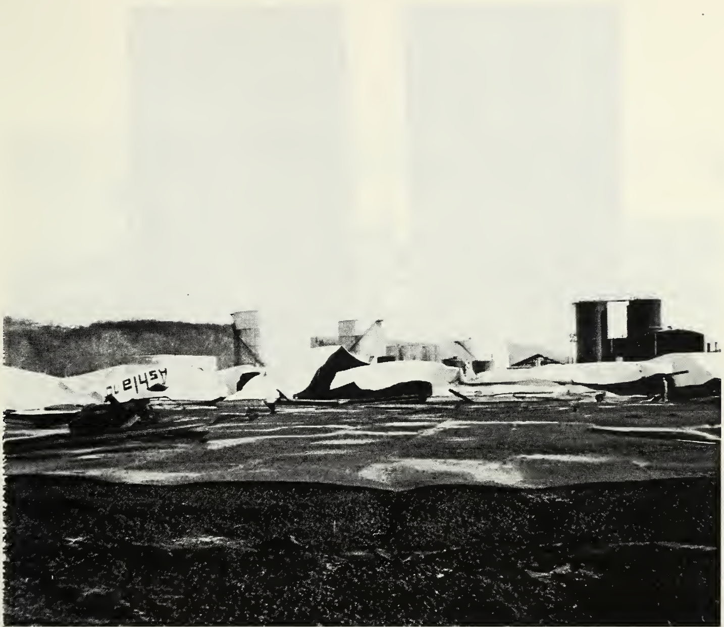
Figure 3.5 - View of Tank Bottom with Tank Wall and Roof in Background
