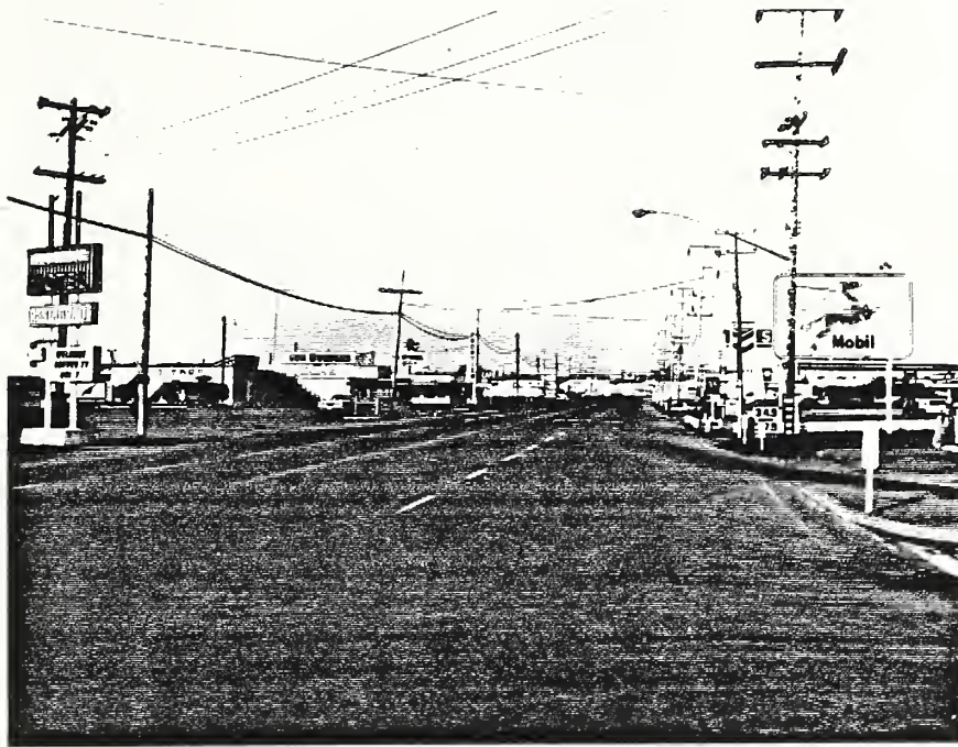
Figure 10a. View of normal conditions at intersection in Crescent City, California.
