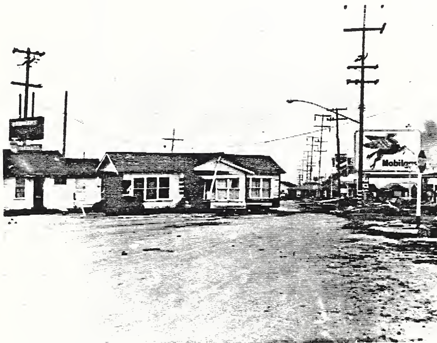
Figure 10b. View of same area as above showing the damage produced by the tsunami generated by the earthquake of March 27, 1964 in the Gulf of Alaska.
