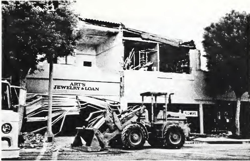
Photo 1 Total collapse of brick masonry wall of 2-story unreinforced masonry building in Uptown, Whittier.
