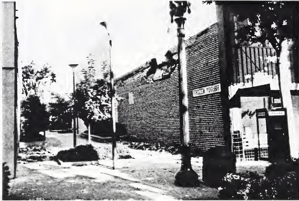
Photo 3 Typical collapse of unreinforced brick wall, Whittier.
