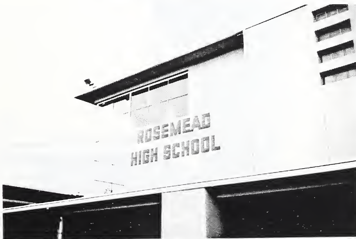
Photo 38 This school building experienced minor structural damage. Note no glass was broken at the corner of the building.
