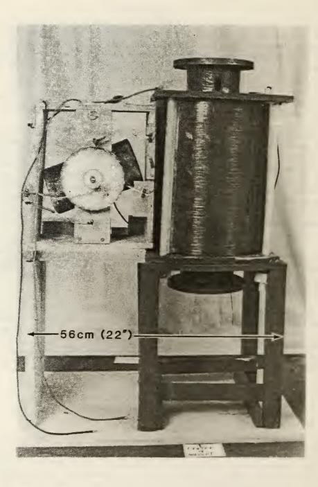
Figure 1. Photograph of Joseph Newman's device which was delivered to the National Bureau of Standards
