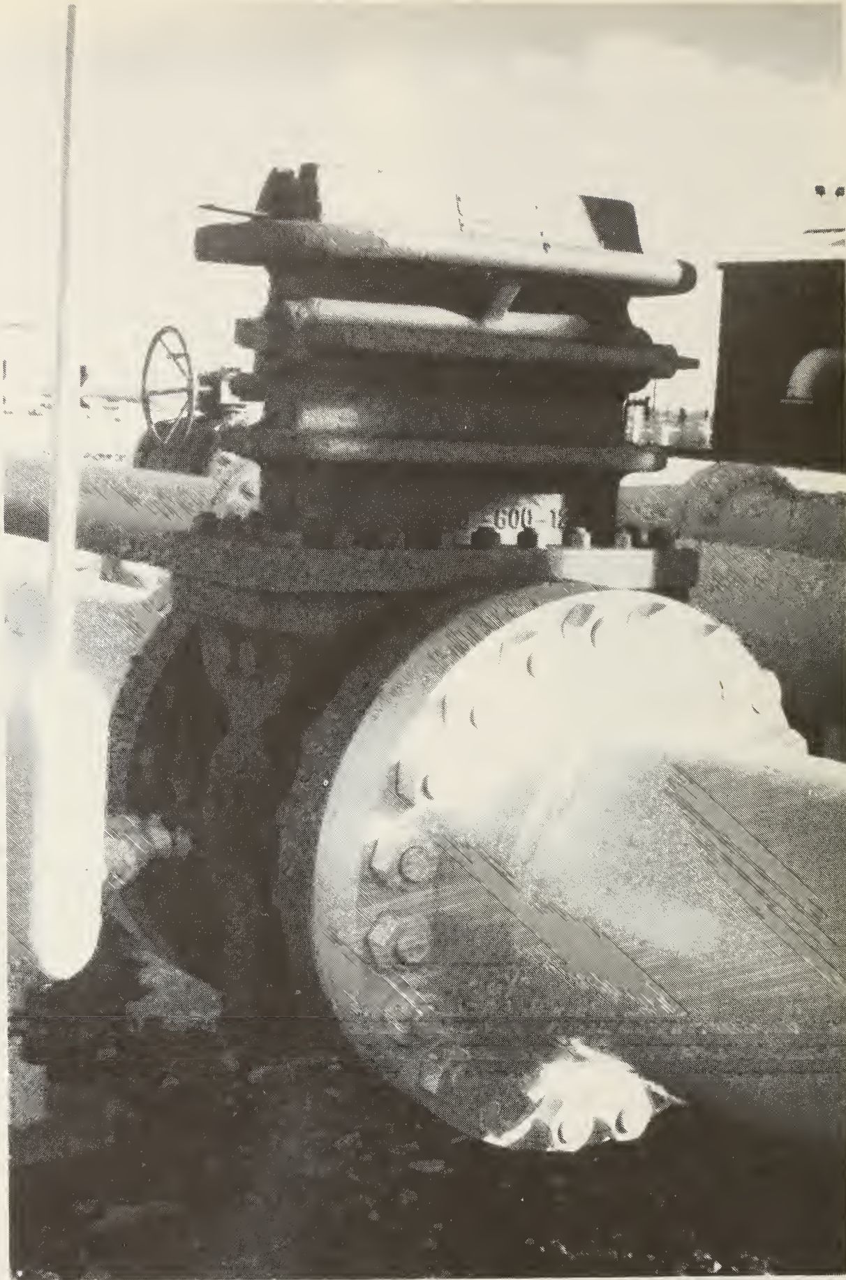
Bonnet type orifice meter fitting
