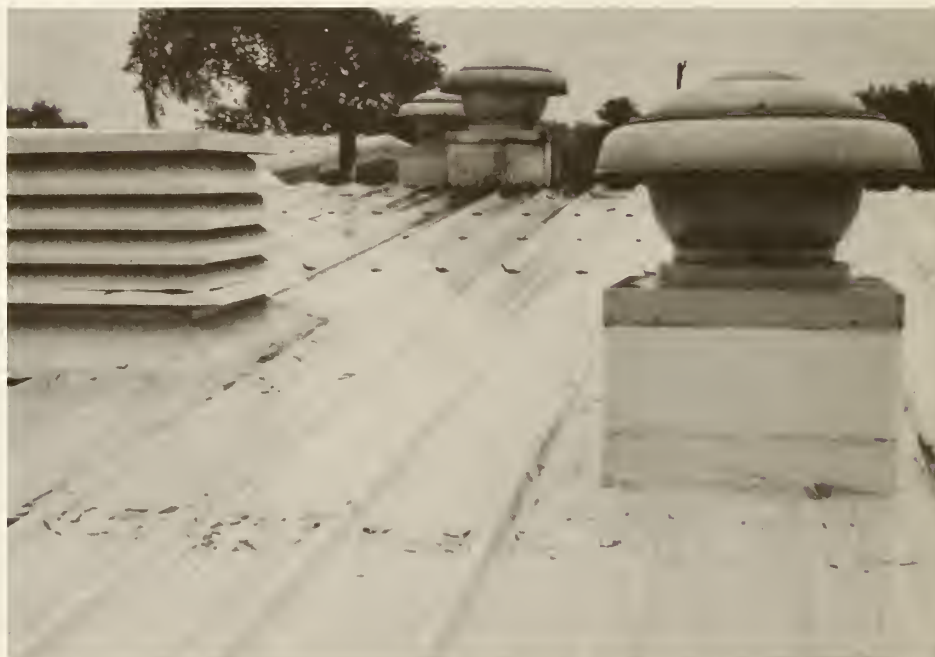
Figure 5. Bituminous mastic material used on roof to cover fasteners
