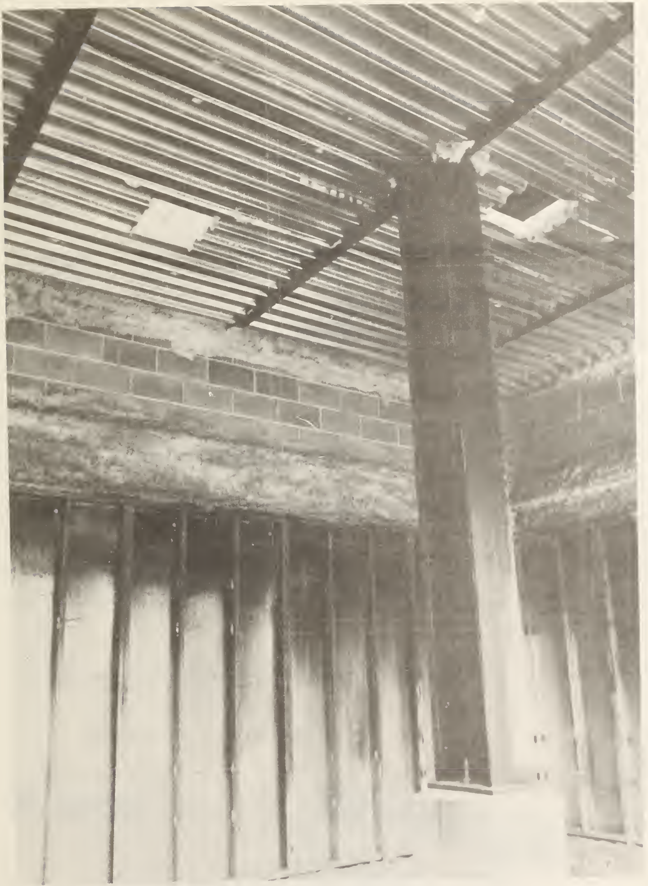
Figure 4. Photograph of fire compartment
