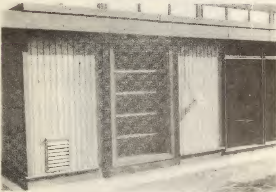
Figure 19. Photograph of vertical aperture with pyranometer installed to right
