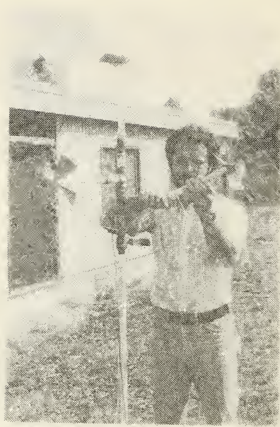
Figure 20. Photograph of three-axis wind sensor installation
