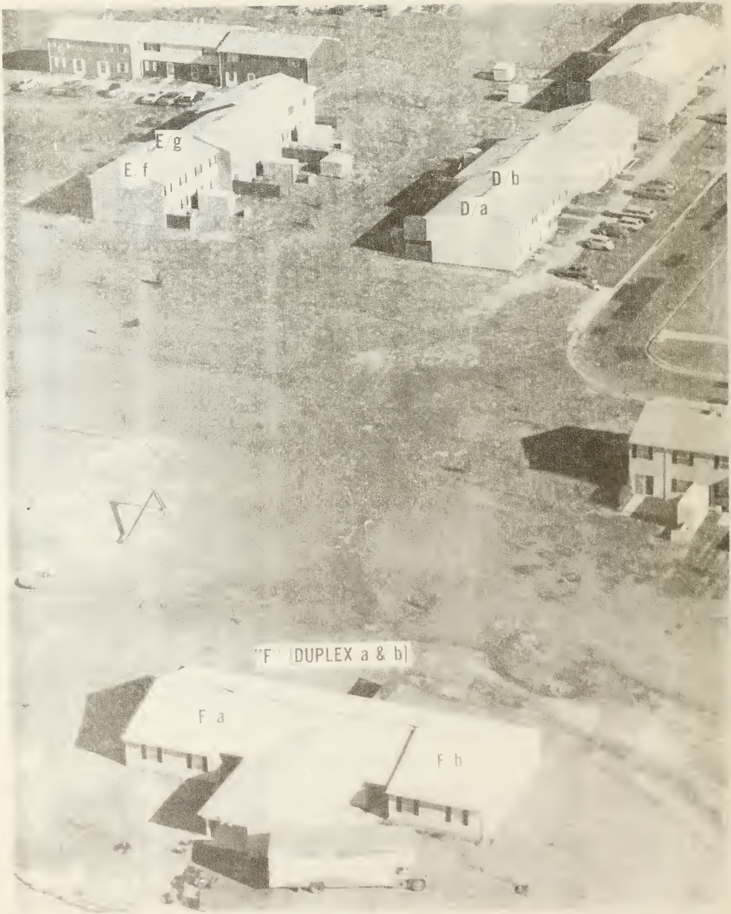
Figure 1. Aerial view of test houses
