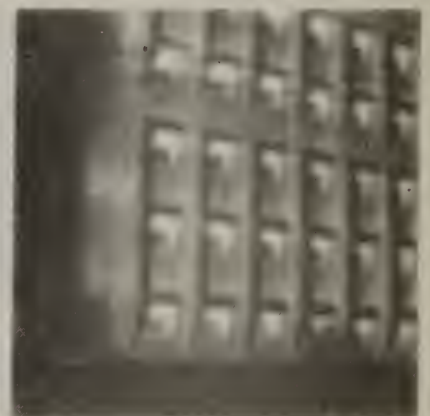
15-4 Lower west face of the tower at the N end
