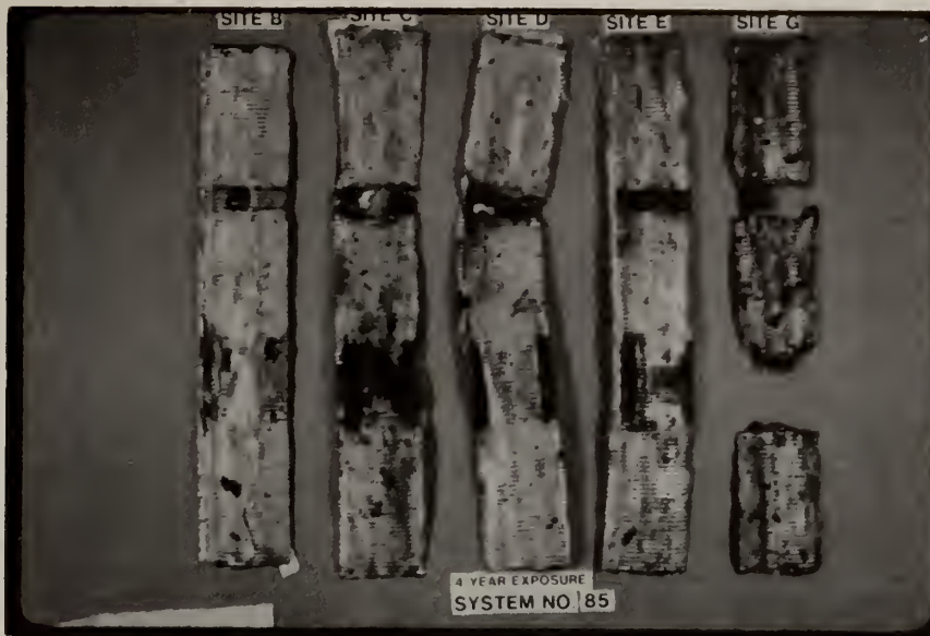
Figure 38. Outer Shield: System 85, Sites B, C, D, E, and G, left to right, exposed for four years. Severe corrosion at the window and ring areas on the specimens from Sites B, C, D, and G.
