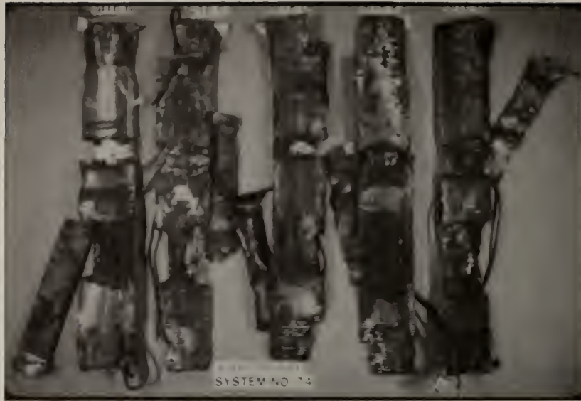
Figure 16. Outer Shield: System 74, Sites B, C, D, E, and G, left to right, exposed for four years. Coupling this system to copper accelerated corrosion on the specimens from all sites.
