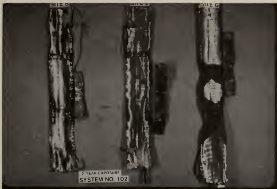
Figure 10. Outer Shield: System 102, Sites, B, E, and G, left to right, exposed for two years. Coupling this system to copper accelerated corrosion on specimens at window and ring areas with severe corrosion on the specimen from Site G.
