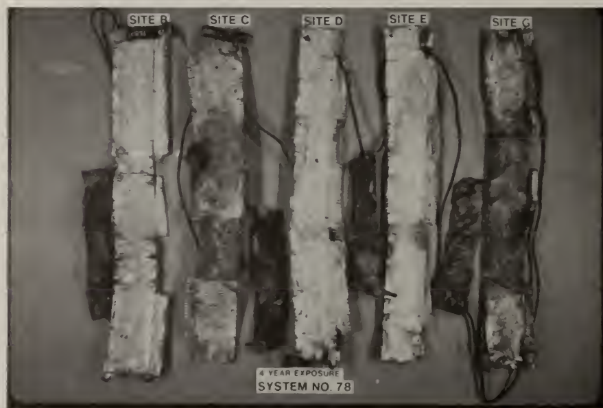
Figure 25. Inner Shield: System 78, Sites B, C, D, E, and G, left to right, exposed for four years. Coupling this system to copper accelerated degradation on specimens from Sites C, E, and G.
