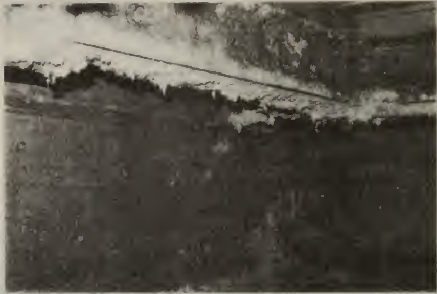
Figure 2.13 Damage to fireproofing due to carelessness while materials were being transported to other areas of the buildings
