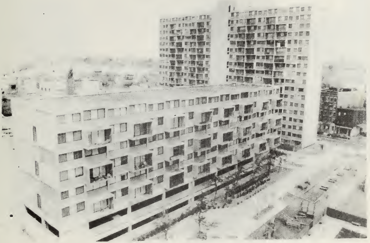
Figure 2.7 Shelley "A" and Shelley "B" buildings
