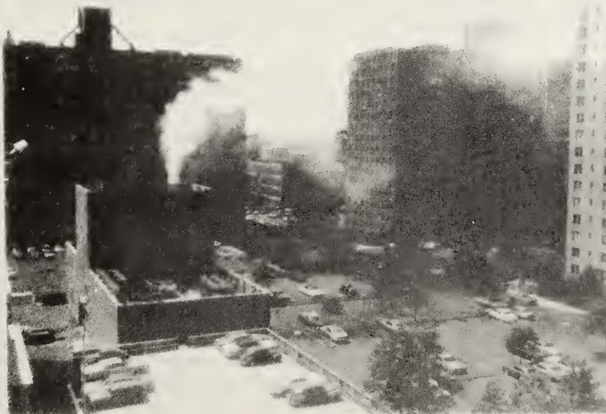
Figure 10.10 Diesel engine exhaust plume with 3-8 mph (1.3 - 3.6 m/s) southerly wind. Visibility of the plume was enhanced by means of a smoke bomb dropped into the stack.
