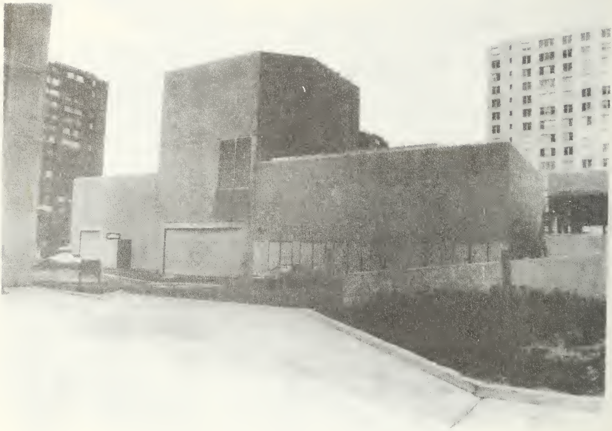
Figure 2.8 Central equipment building
