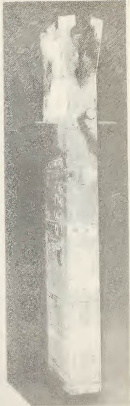
d. Top of box beam segment 9M (NBS 3-5).
