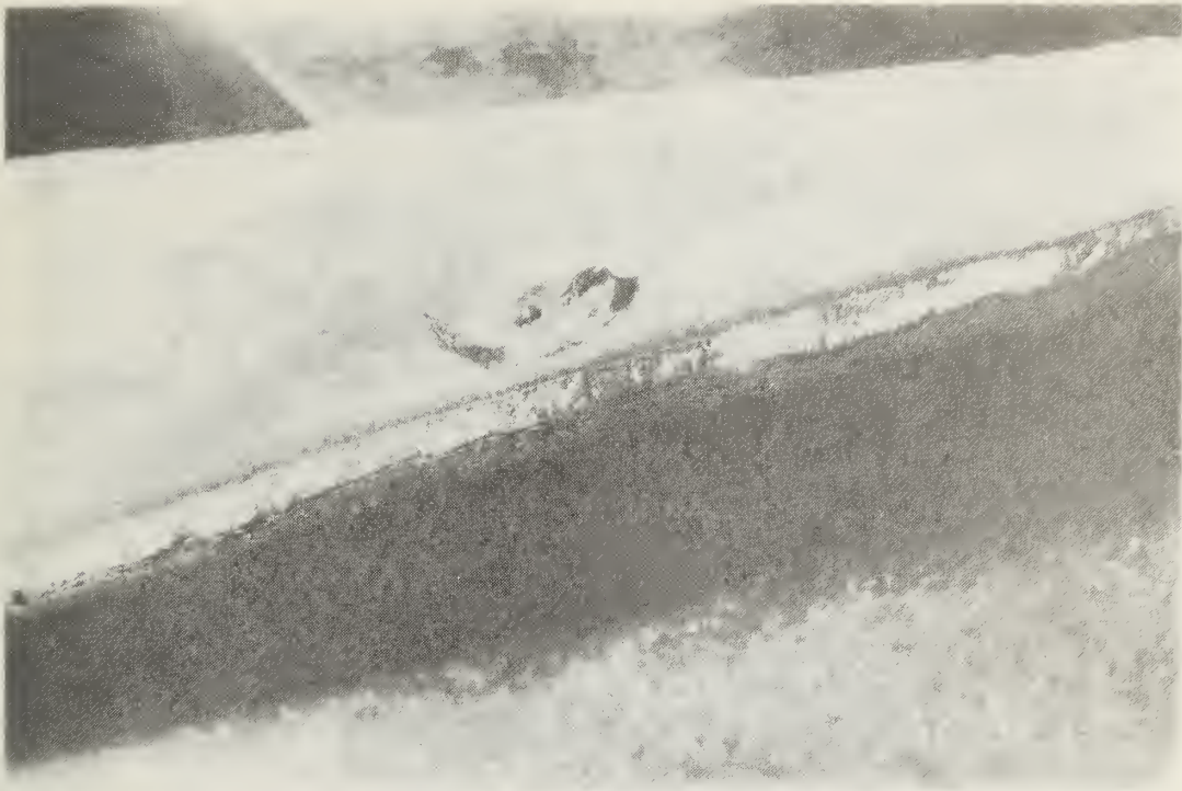
Figure 5.15 Weld penetration at location 8UW, upper flange.
