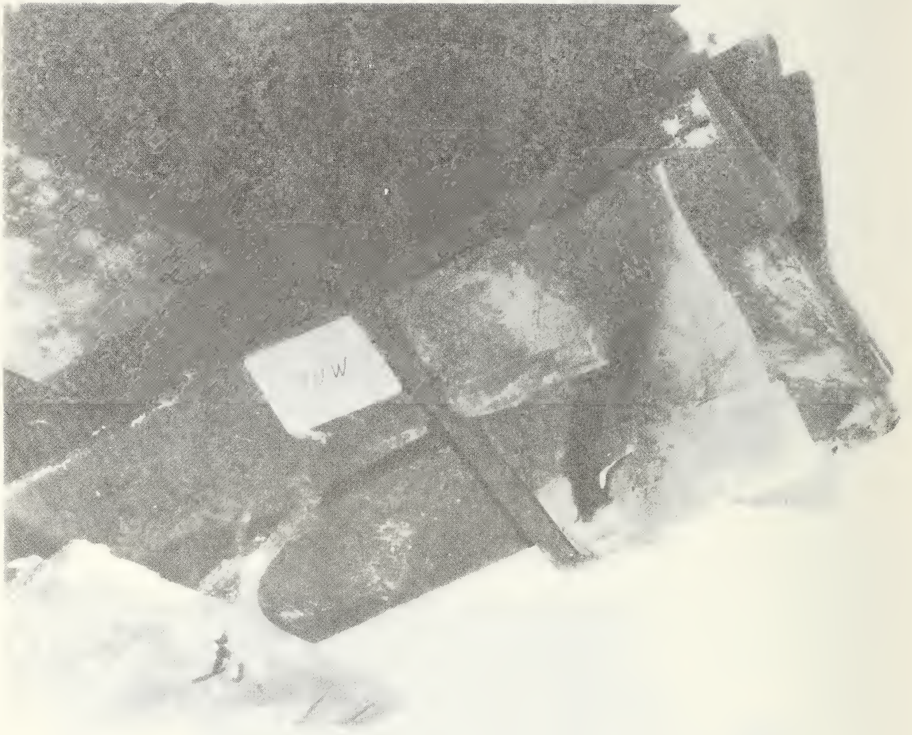
Figure 5.27 Modified bearing pad at location 11UW.
