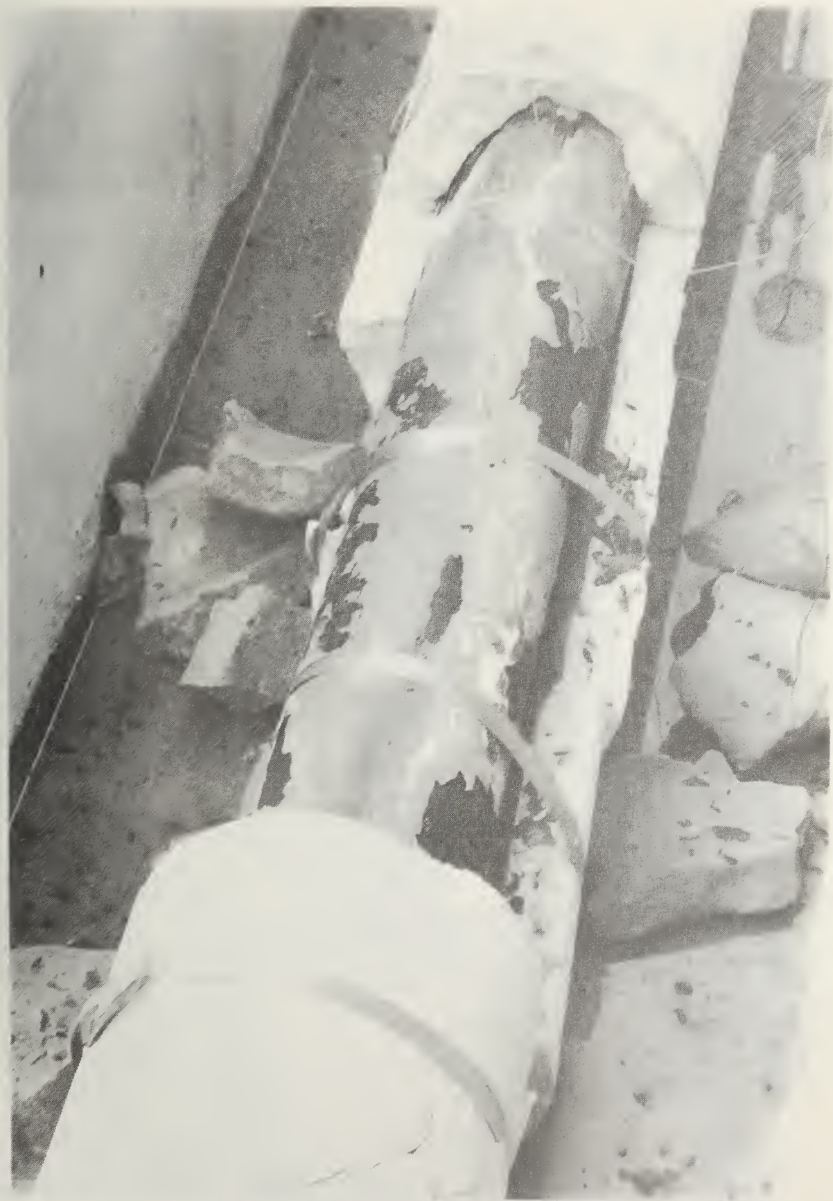
Figure 9. Kaylo #2 system after 72 hours boiling and 24 hours drying.
