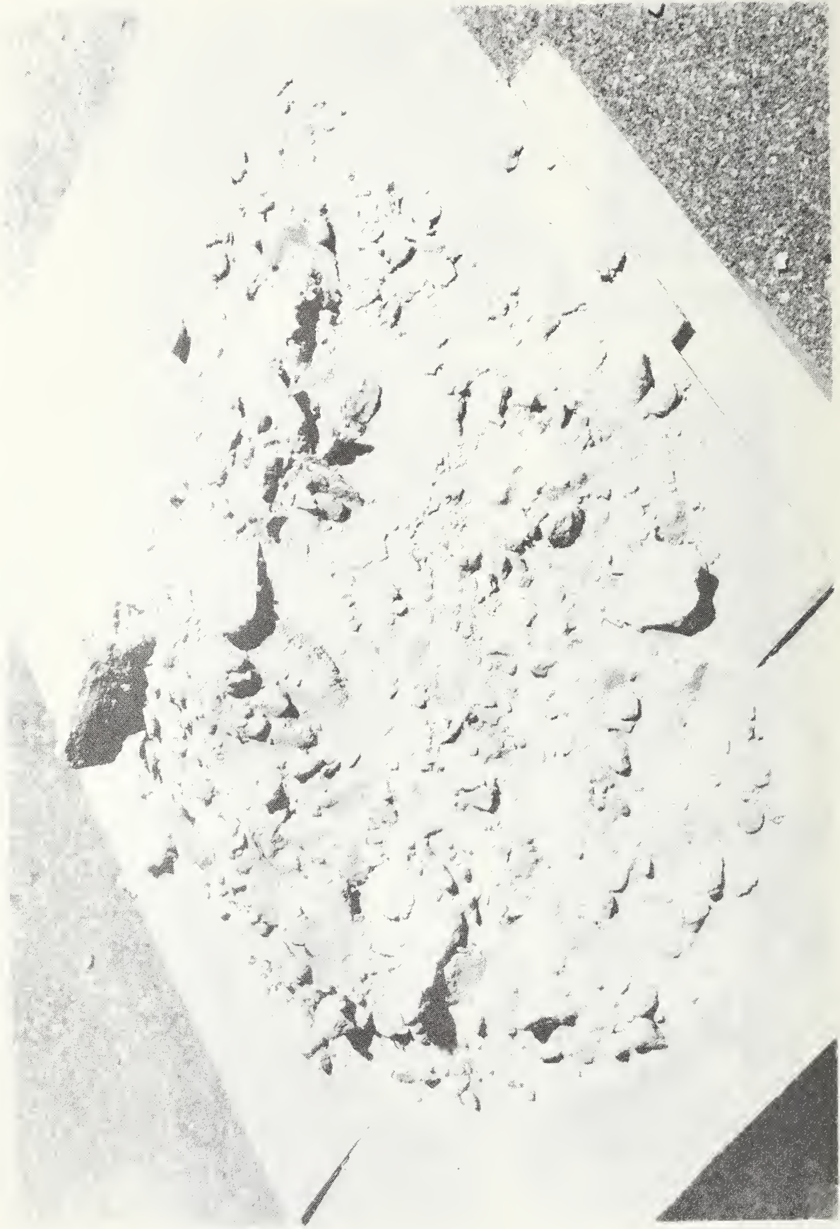
Figure 60. Crumbs of insulation found in the conduit space after the carrier pipe and insulation jacket were removed (Celotemp system).
