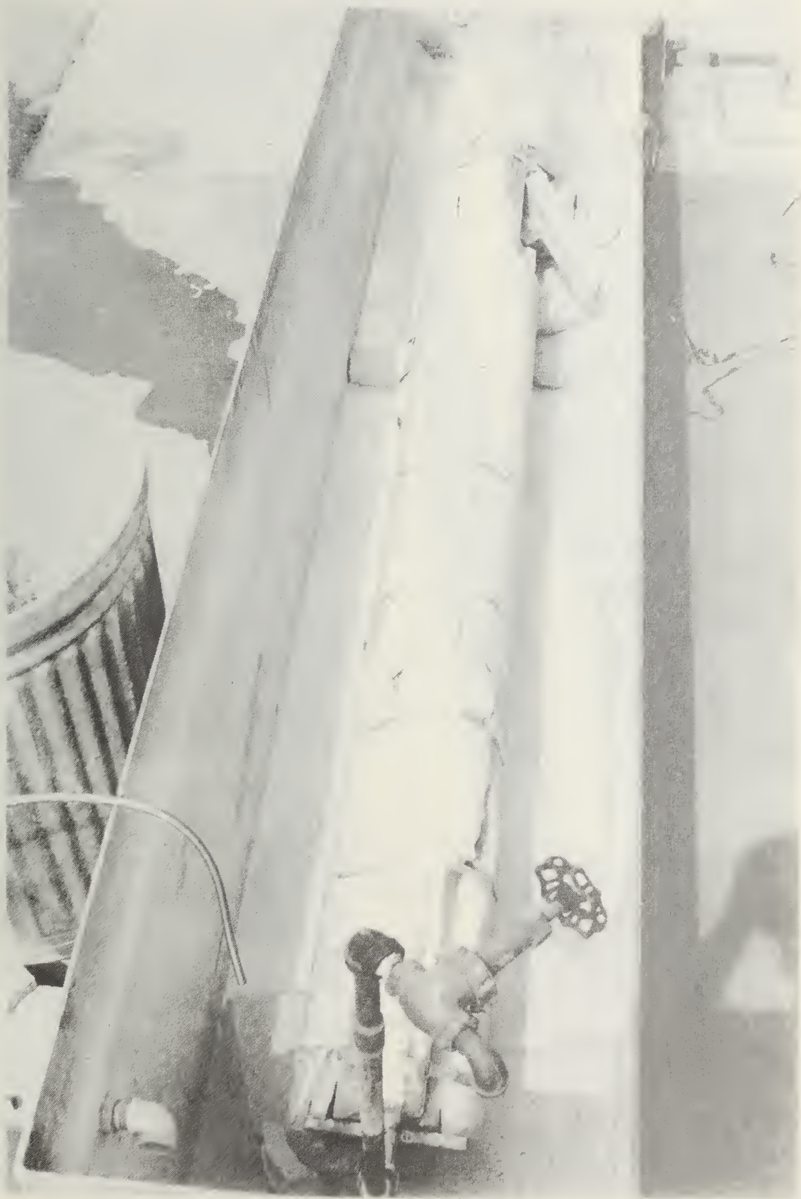
Figure 19. PABCO #2 system after 3 hours boiling
