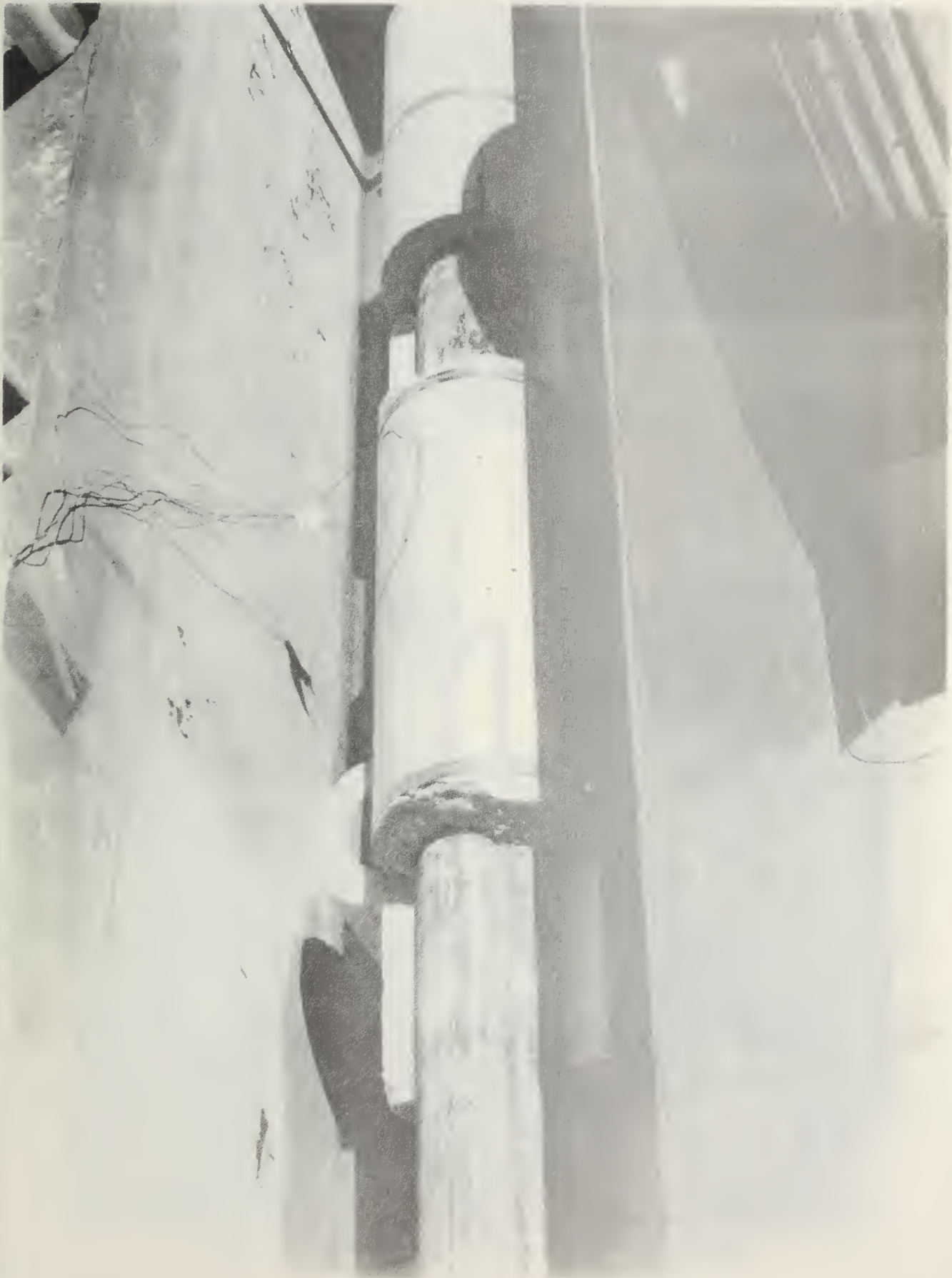
Figure 15. PABCO #1 system after 1 hour boiling
