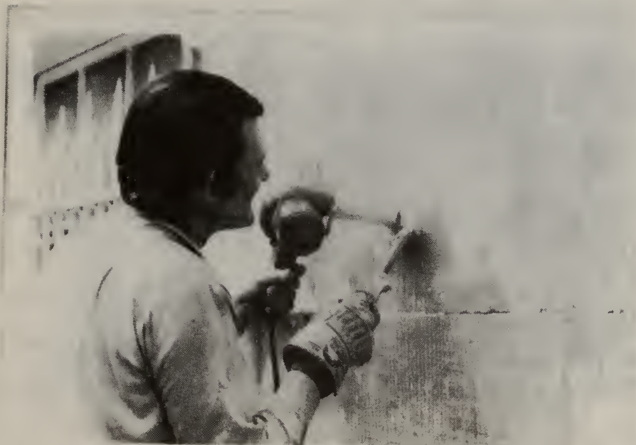
FIGURE 22. PAINT REMOVAL IN AREA A, USING HIGH PRESSURE WATER SPRAY
