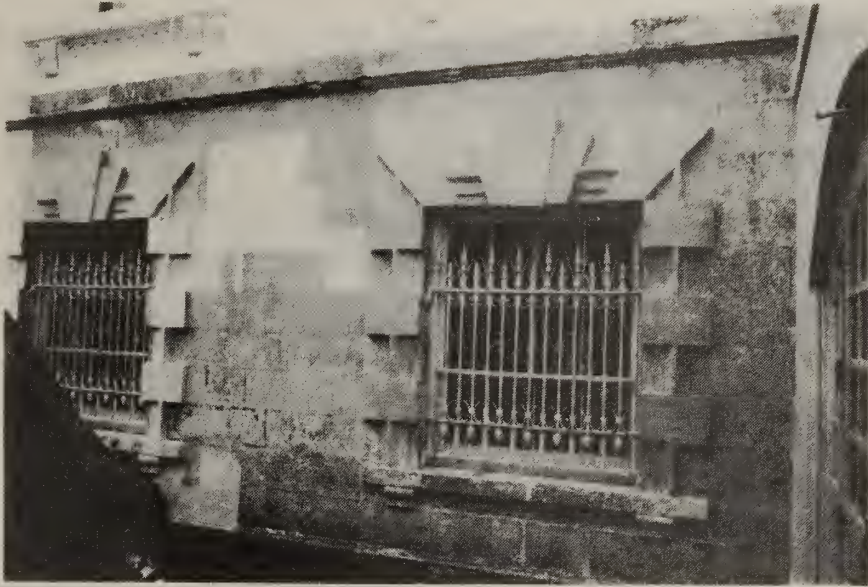
FIGURE 34. AREA D, WITH MOST OF THE PAINT REMOVED
