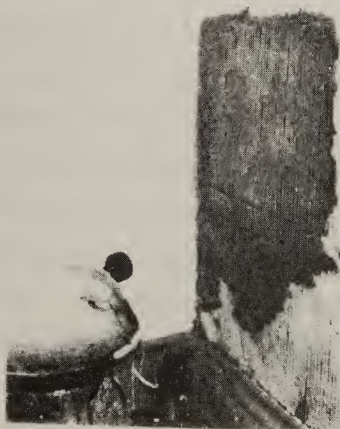
FIGURE 36. AREA A, REPAIRED AREA
