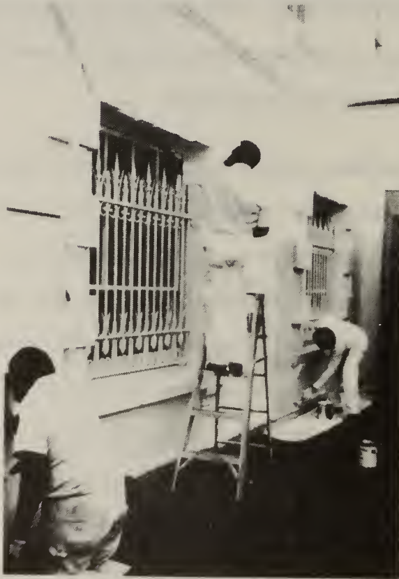
FIGURE 39. REPAINTING OF AREA D
