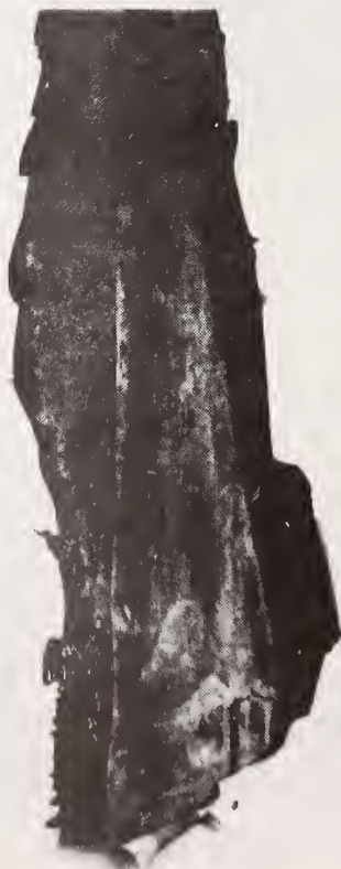
Figure 21 -- Nose Dock, MacDill AFB, Delamination of Elastomeric Coating (see Figure 20).
