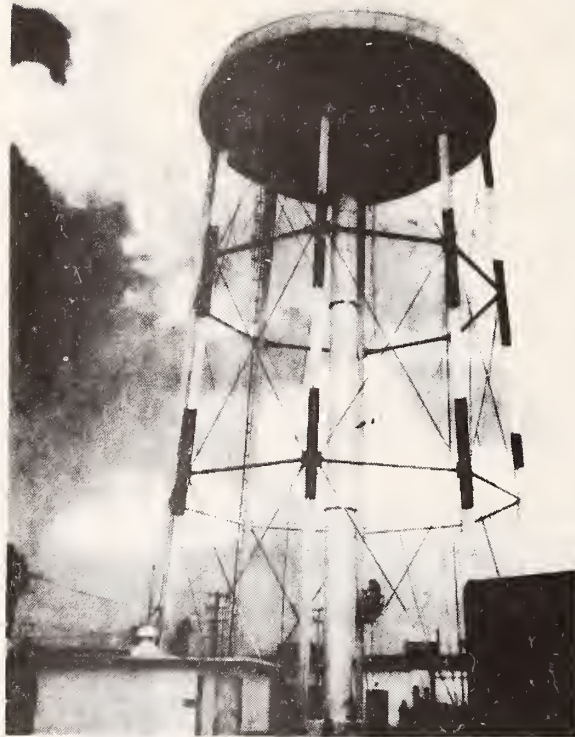
Figure 8 -- Water Tower, Patrick AFB, Overall View of Tower Undergoing Repair.
