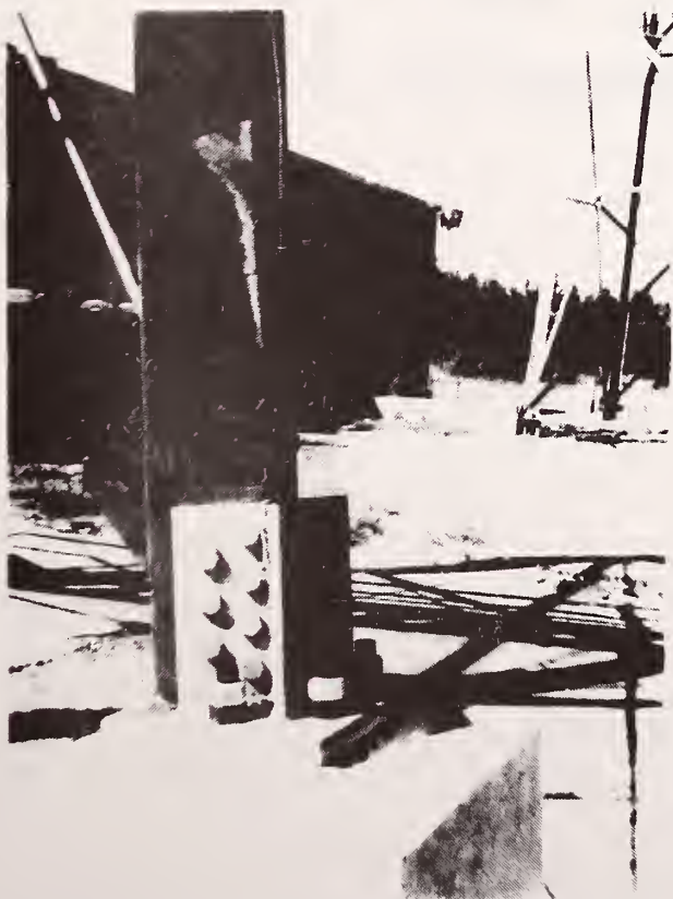
Figure 35 -- Communication Tower, Tyndall AFB.
