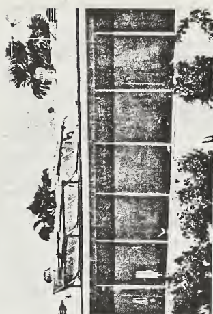
"Concentrating" type solar collectors use a trough shaped mirror to collect solar energy and tracks the sun as it moves across the sky.
