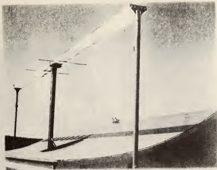
Figure 2-30. Concentrating Collector with Roof Mounted Reflective Surfaces
