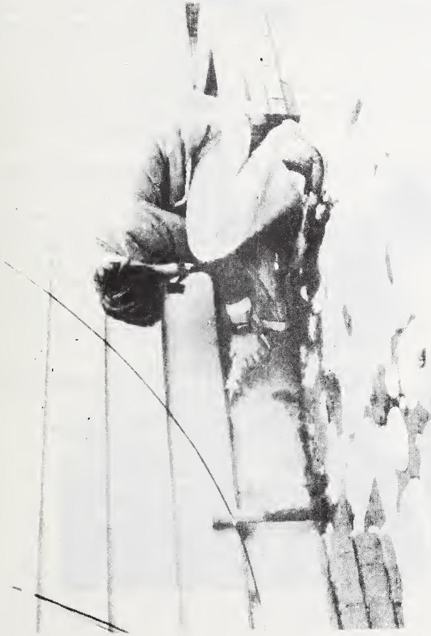
Figure 4. Caulking compound being applied to foundation sill.
