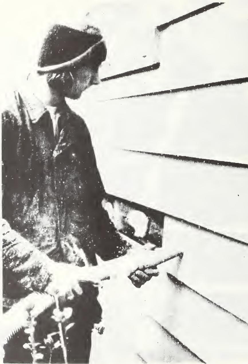
Figure A-3. Cellulosic fiber being blown into the walls of the test house.
