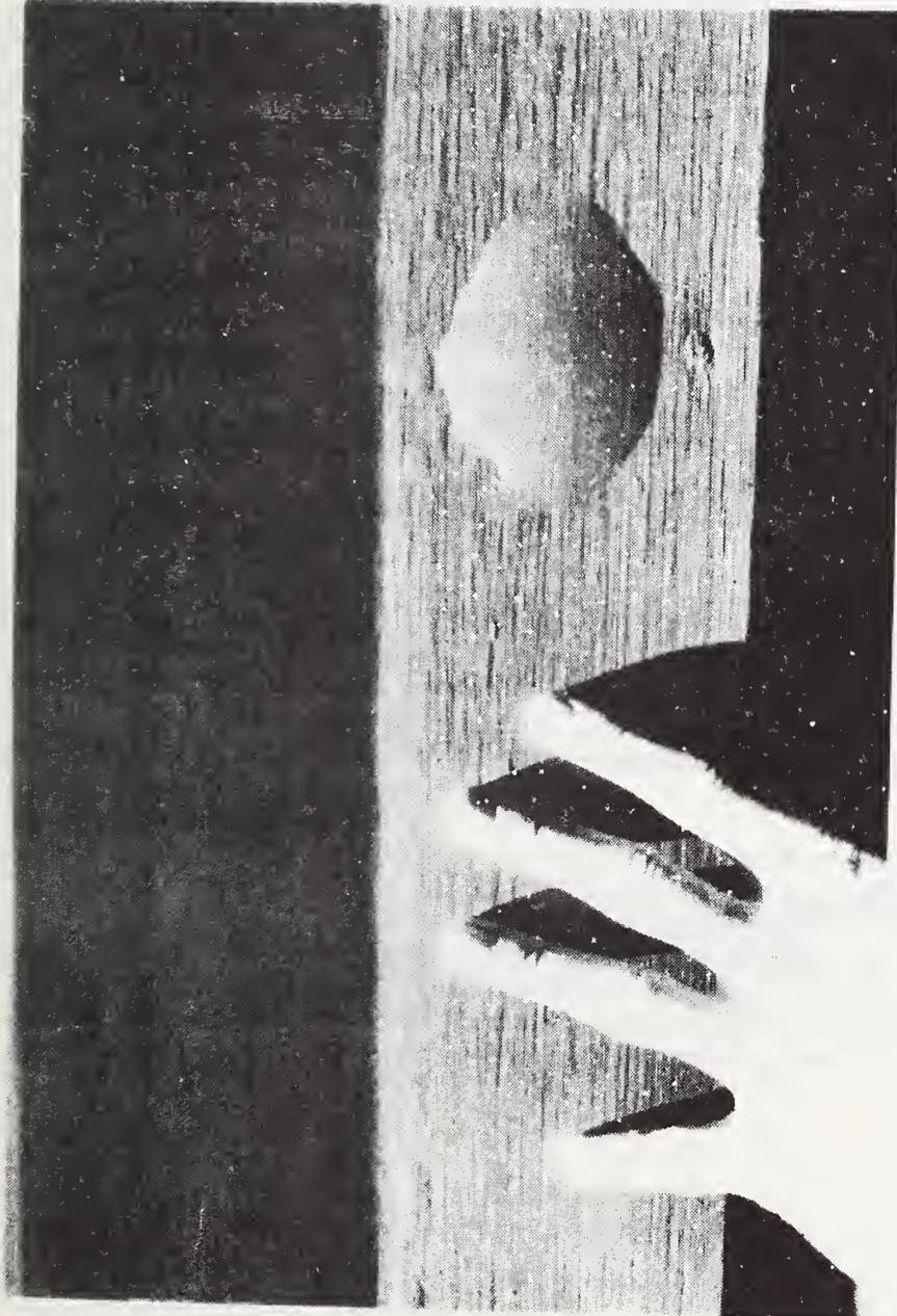
Figure 32. Water blister at exterior surface of U-F wall section.
