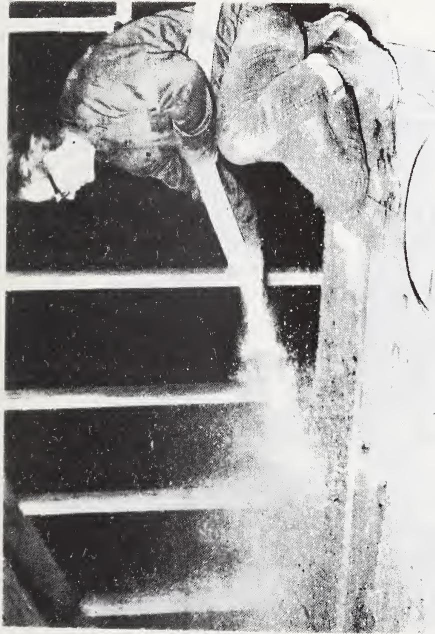
Figure A-2. Loose-fill cellulose being blown on top of the existing ceiling insulation.
