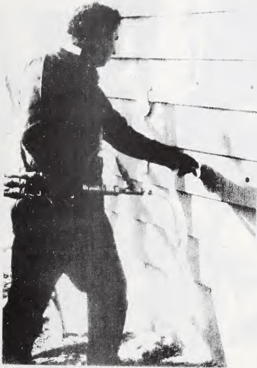
Figure A-5. Urea-formaldehyde foam being blown into a wall section.
