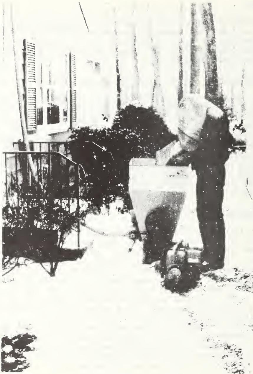
Figure A-1. Loose-fill cellulose insulation being poured into blowing machine.
