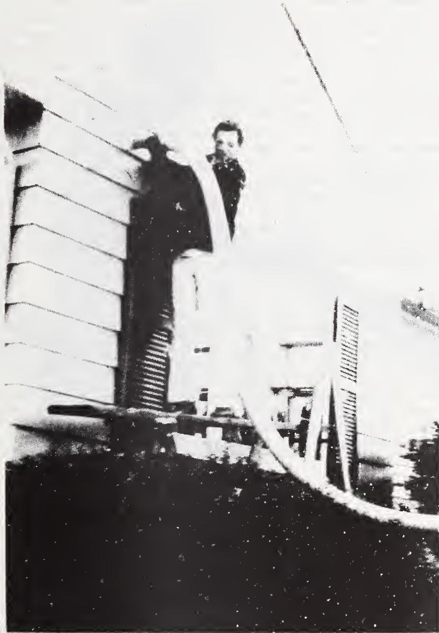
Figure A-4. Glass fiber being blown into a wall section.
