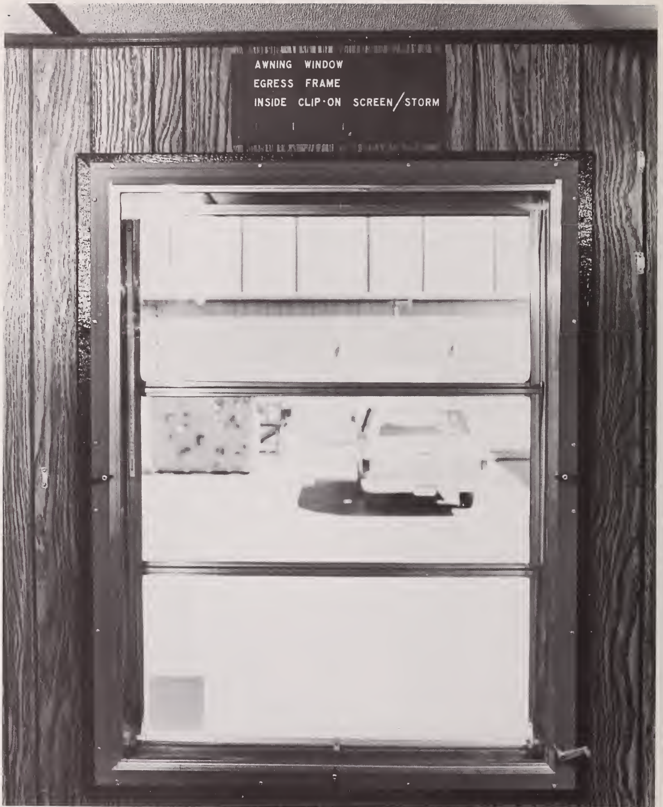
Figure 3. Demonstration Unit. Awning window in egress frame
