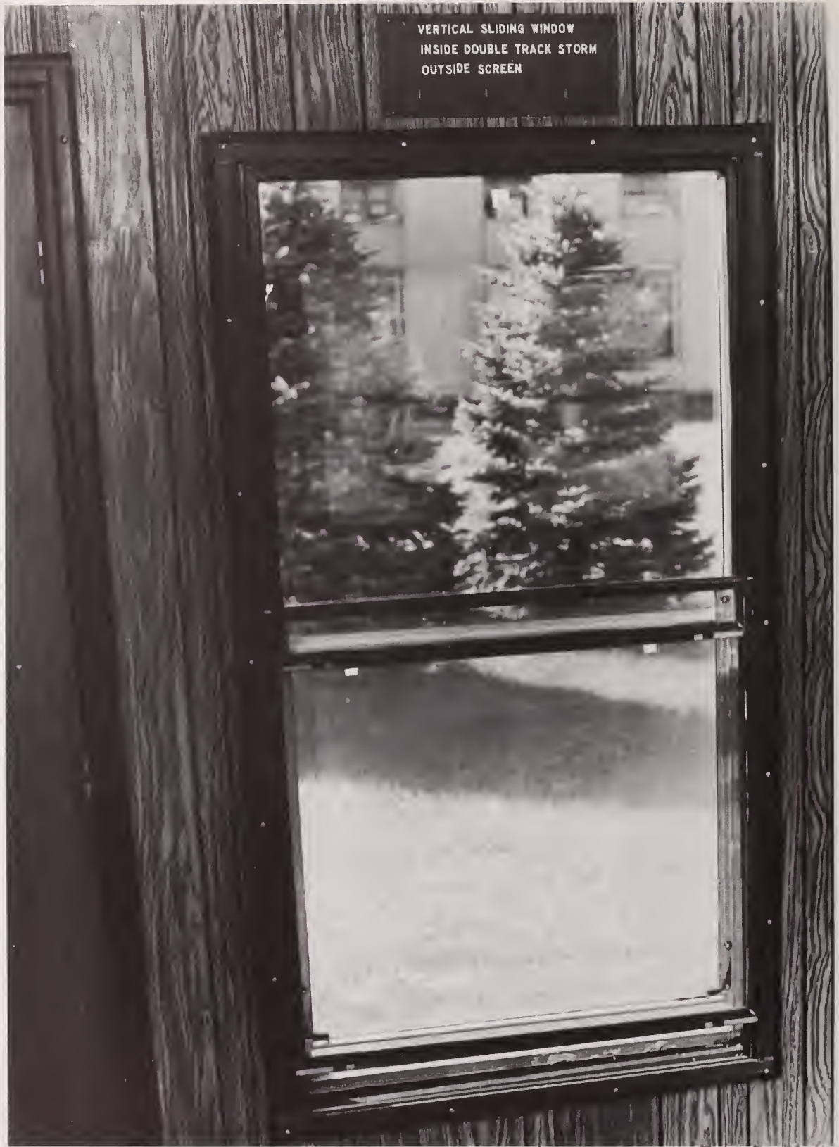
Figure 7. Demonstration Unit. Vertical sliding window
