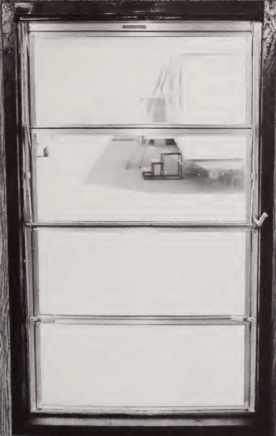
Figure 6. Demonstration Unit. Pop-out awning window
