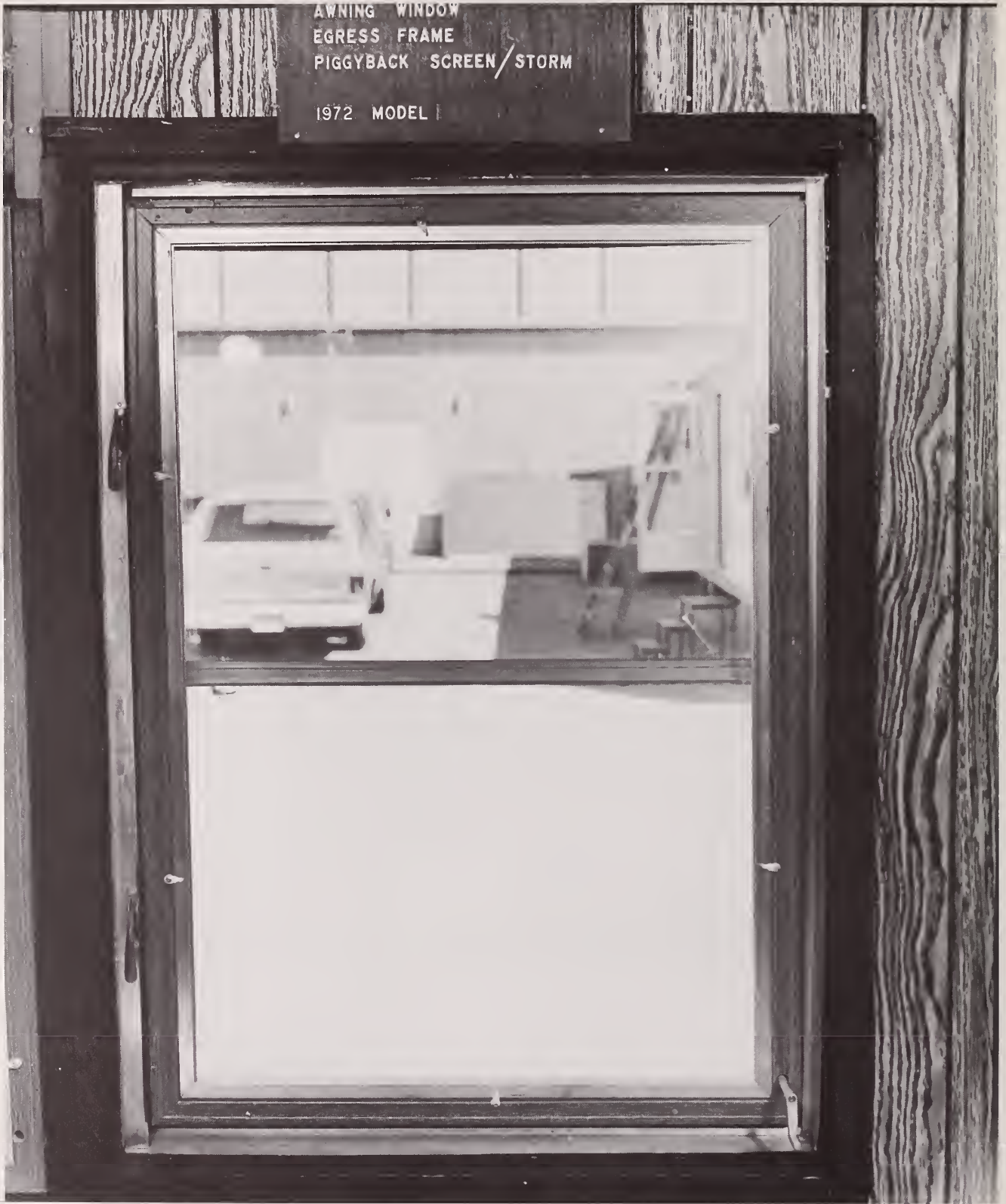
Figure 9. Demonstration Unit. Awning window in piggyback egress frame
