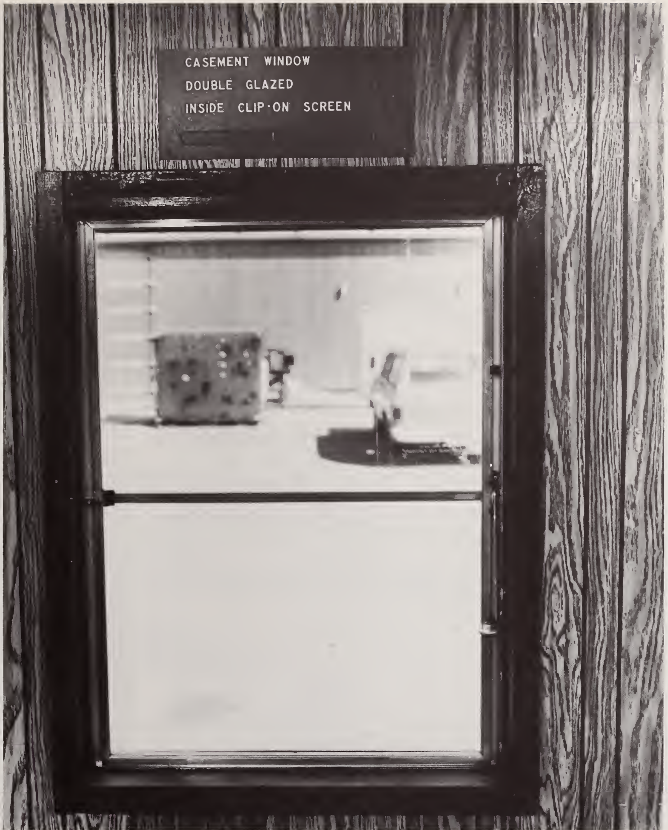
Figure 2. Demonstration Unit. Casement window
