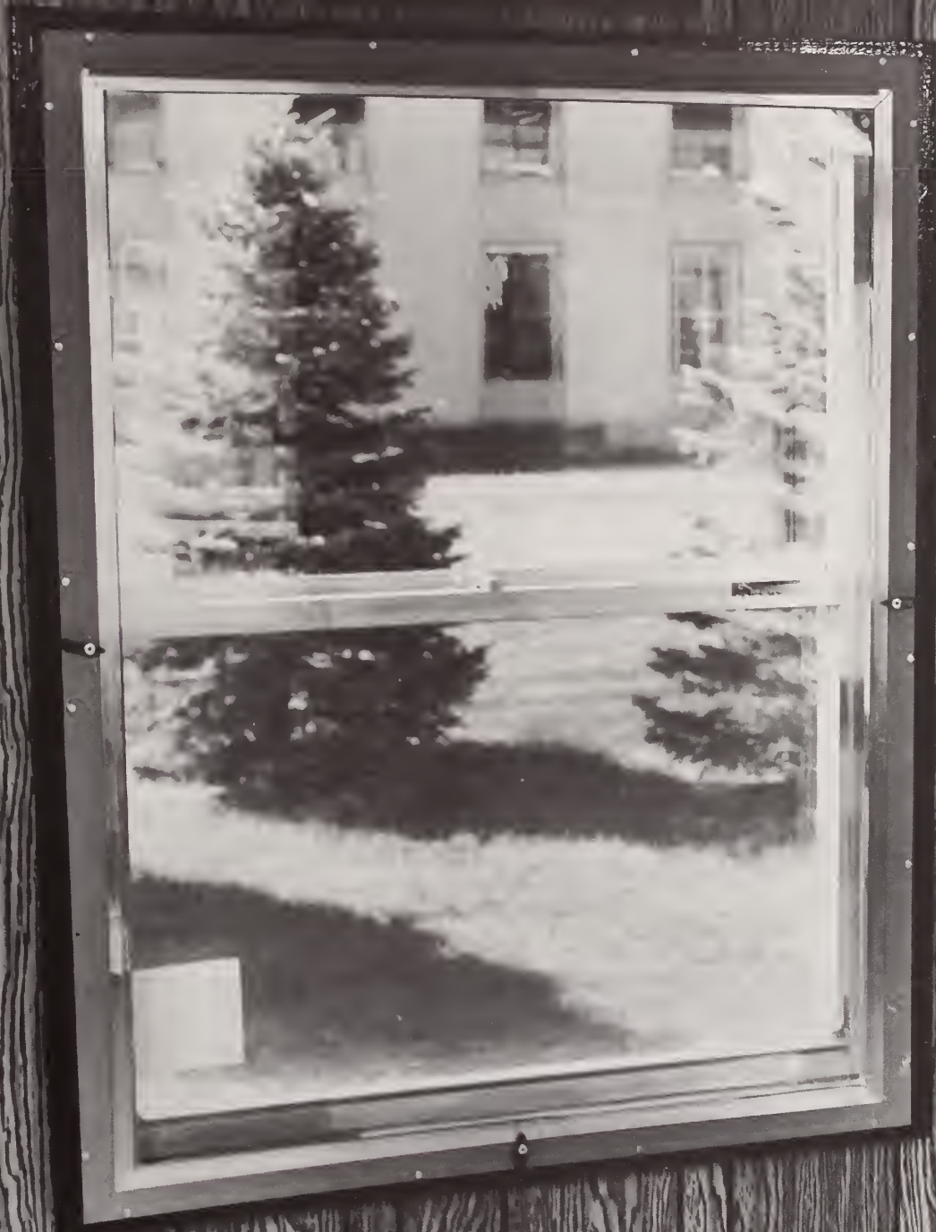
Figure 4. Demonstration Unit. Vertical sliding window in egress frame
