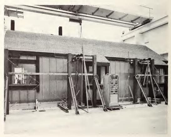
Static and dynamic testing is accomplished by use of a heavily reinforced tie-down floor permitting mounting of complete structural members. Hydraulic actuators provide test loads in dynamic tests. Automatic recording of up to 200 channels of sensor data is accomplished by a mini-computer-controlled data acquisition system.
