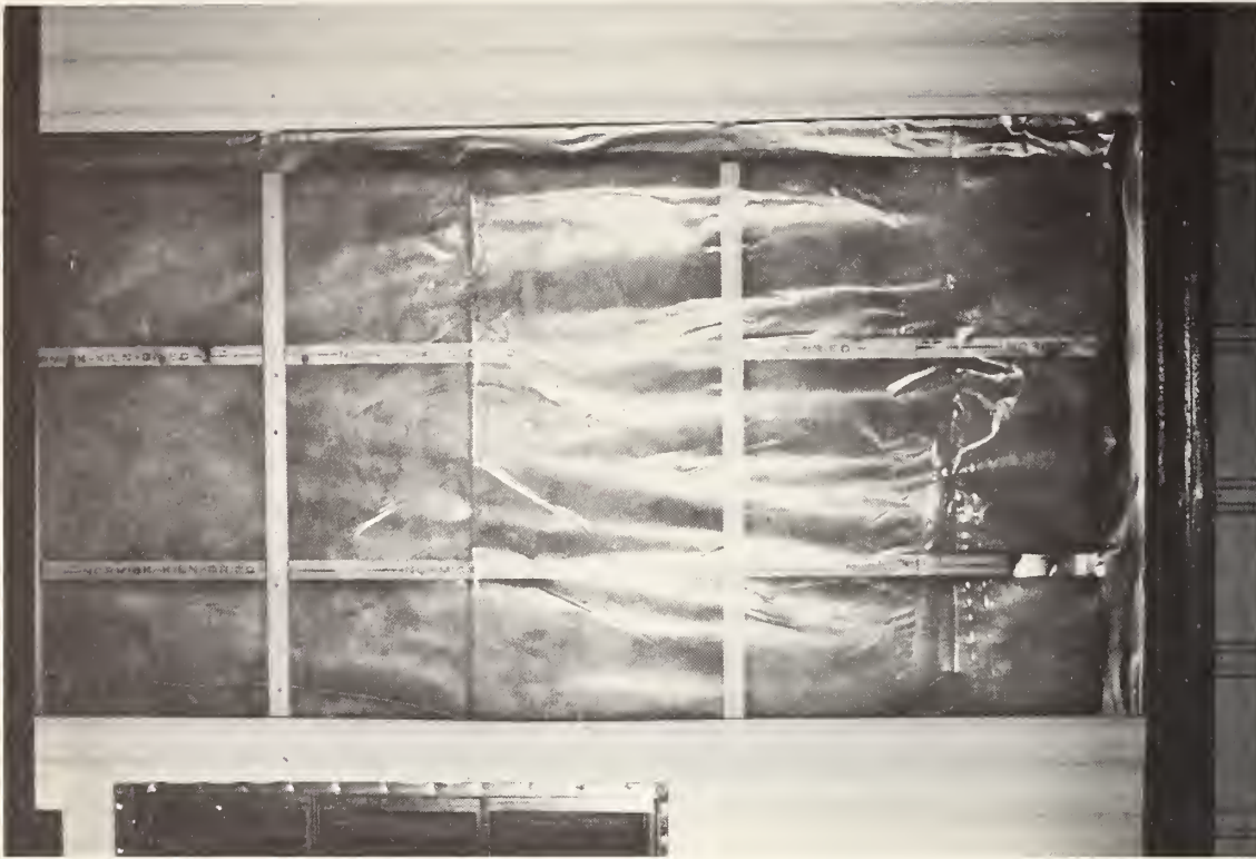
Figure 33. Six mil. polyethylene film used to seal insulation cavity from penetration of outside air.
