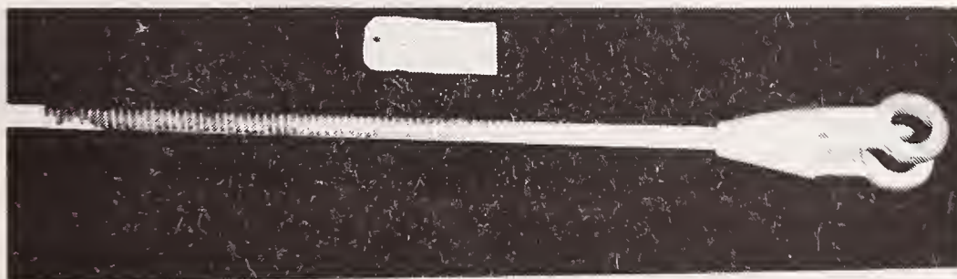
Figure 6. Upper end of Rod X4 showing substantial loss of coating. The helical markings on the uncoated surface are clearly visible.
