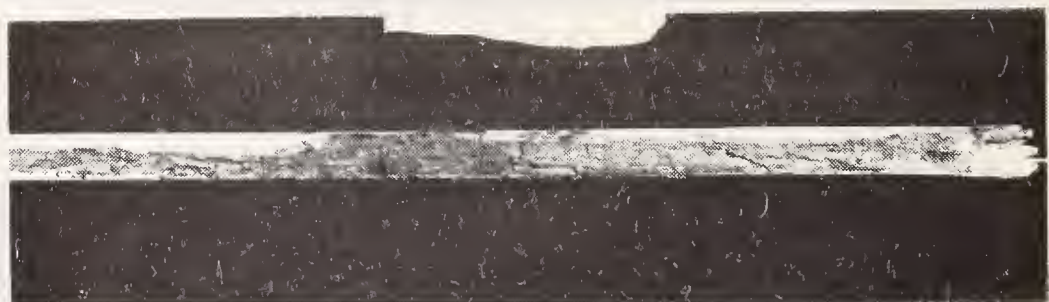
Figure 10. Upper end of Rod X8 showing severe carbonaceous tracking and charring. The rod appeared to have burned almost completely through, with the last 3 percent of its cross section having failed in tension. Some small areas of coating loss are evident along the upper edge of the burn damage. The fitting from this end of the rod is shown in Figure 20.
