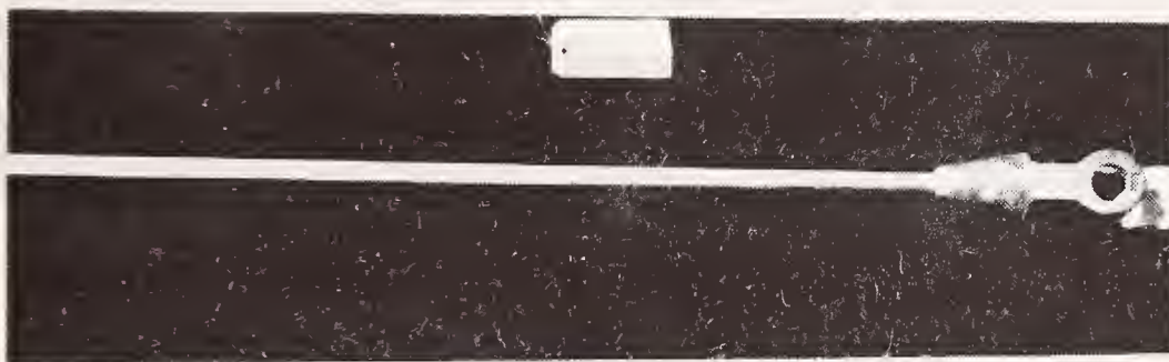
Figure 5. Upper end of Rod X3 showing substantial loss of coating. Helical markings are faintly visible on the uncoated surface.
