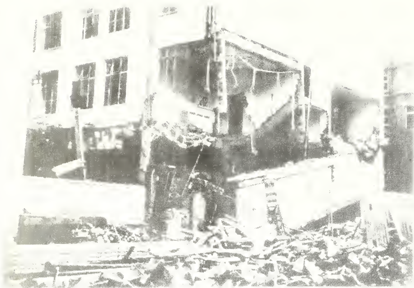
Figure 2 Detail of a Seven-Story-Steel-Framed Building After a Wartime (World War II) Bomb.
