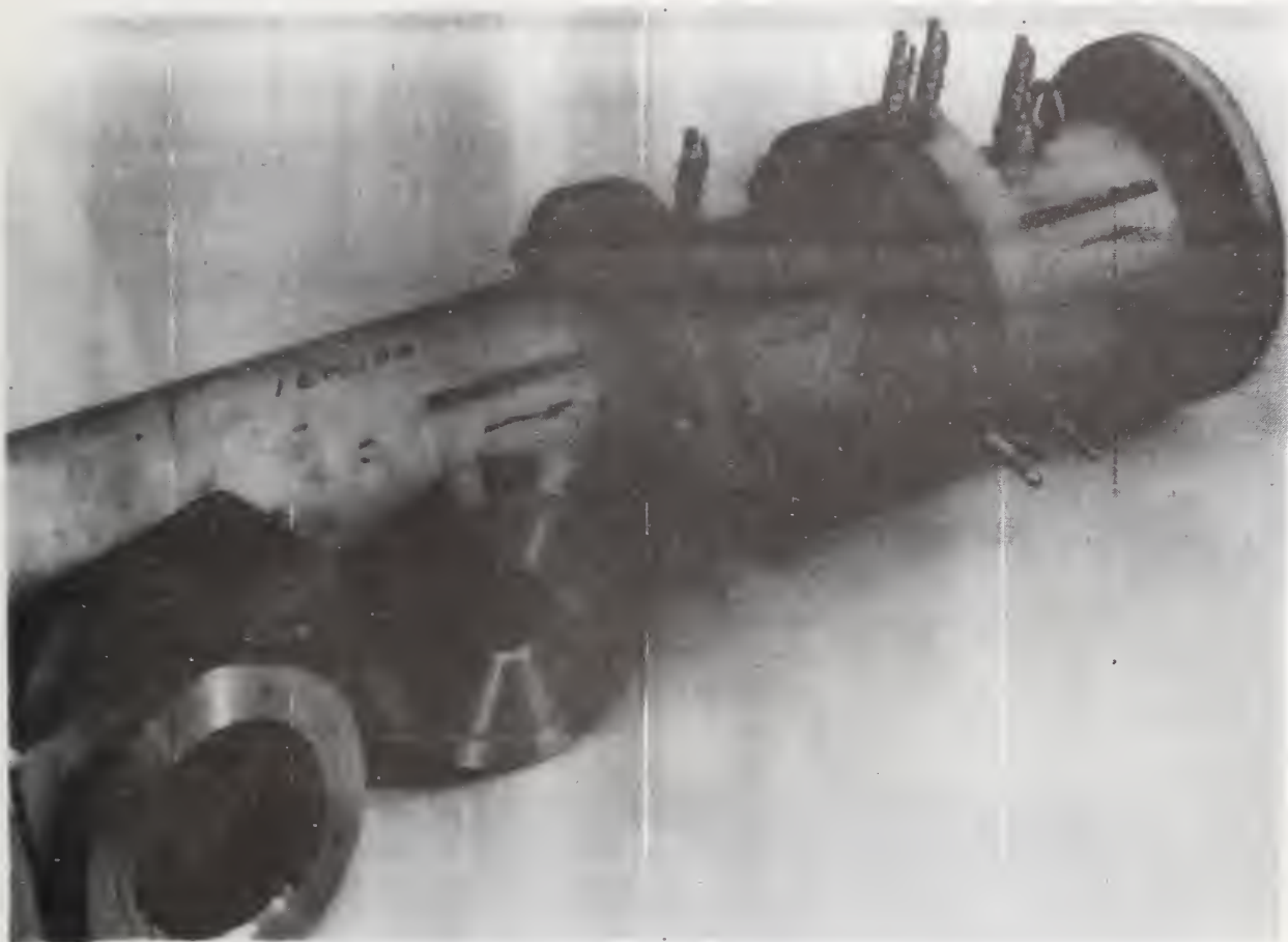
a. Orifice meter run and orifice plates
