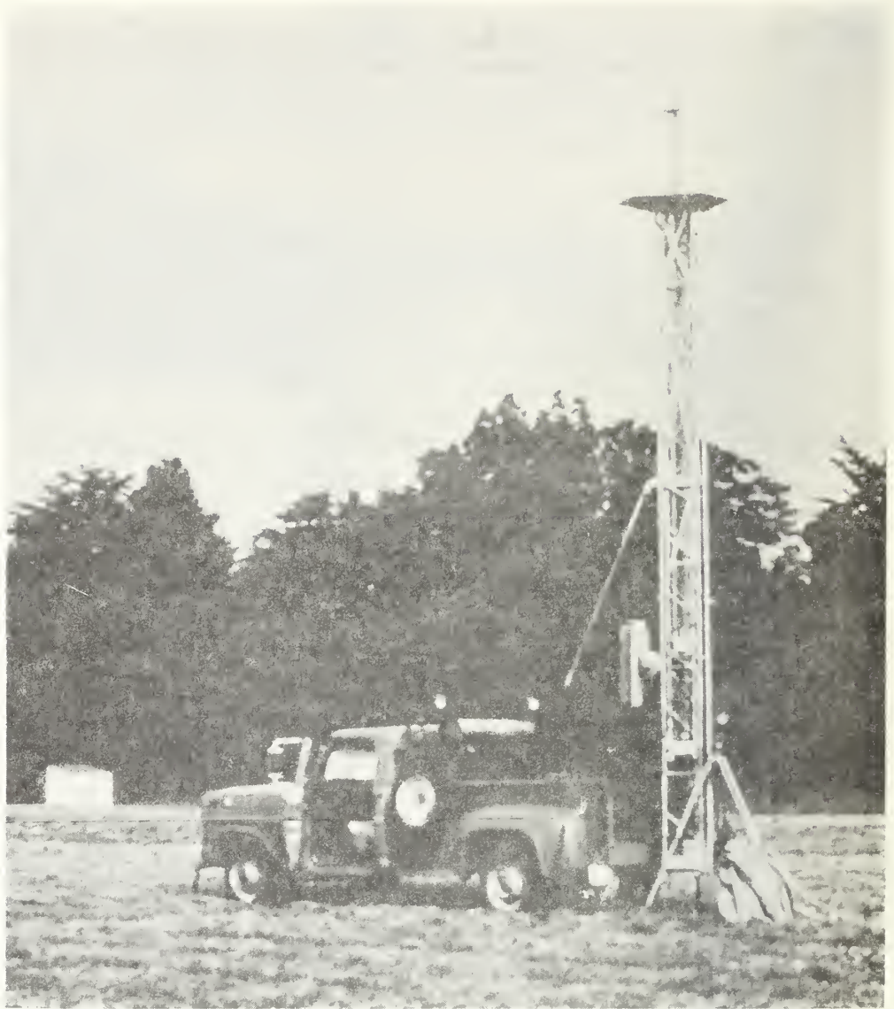
Electronic Distance Measurements from a Portable Tower.
