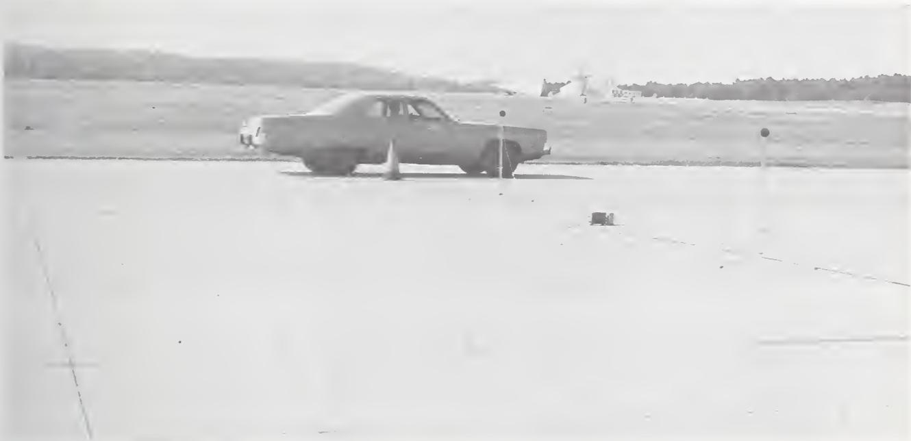
Figure 12. Overall view of the microphone array with the test vehicle (concrete test section, Wallops Station site). The array consisted of two tripod-mounted microphones located at 25 and 50 feet (7.6 and 15.2 m) from the centerline of vehicle travel along a line perpendicular to the vehicle path.
